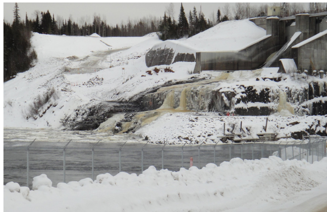
Figure 4 – Kipling access road and marine pad construction was completed.
