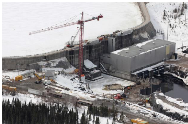
Figure 5 – Little Long shore tie-in construction continues with grout injection required to complete the shore tie-in abutment.
