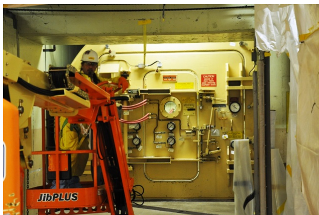
Figure 16 – A worker moves a snorkel lift away from the equipment airlock in unit 1. A project to upgrade airlocks and transfer chambers in unit 1 was recently announced complete.
