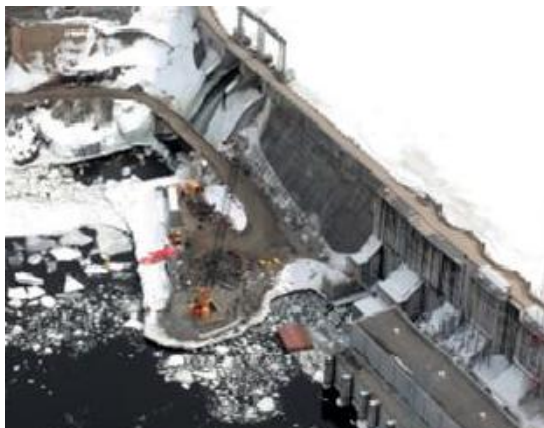
Figure 3 – The crawler crane was mobilized to site and ready for cofferdam installation.
