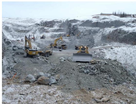
Figure 6 – The Smoky Falls earth cofferdam dewatering is complete. Excavation continues for powerhouse, intake and tailrace footprints.
