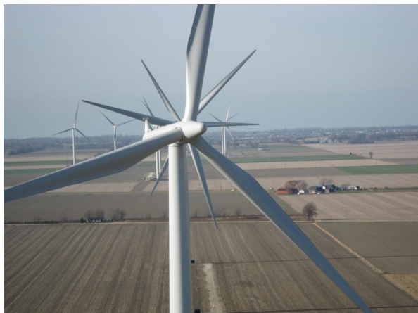
Figure 9 – Kruger Energy Chatham Wind Project achieved commercial operation on January 1.
