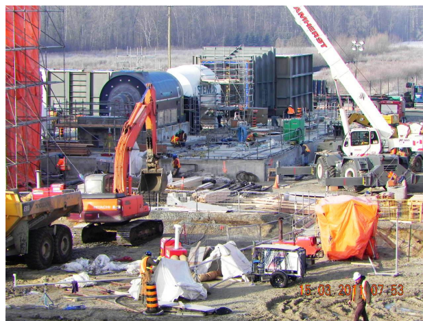
Figure 14 – Mobilization of natural gas pipeline connection contractor to site is in progress. Hydro One has begun construction of the support towers for the 230-kV interconnection on the Hydro One right of way.
