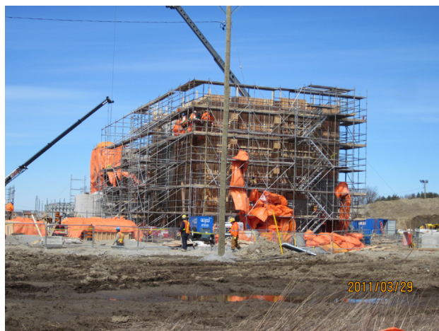
Figure 13 – Foundations for unit #1 and #2 turbines and generators were completed and both units set in place.
