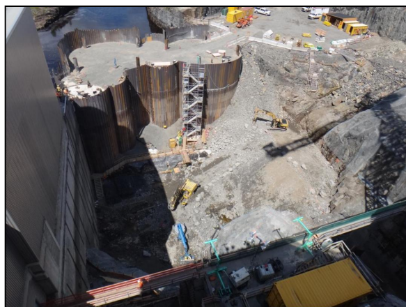
Figure 7 – Little Long cofferdam was completed successfully. Drilling and blasting for rock removal is nearly complete, and preparatory work for concrete pouring is underway.
