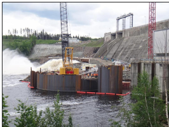
Figure 5 – Harmon cofferdam cell #1 construction is complete and installation of cell #2 is in progress.
