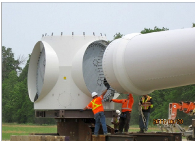
Figure 1 – Workers installing one of the three turbine blades to a rotor hub. Siemens-manufactured turbine components including nacelles, rotor hubs, blades and towers started arriving at the project site. The towers were manufactured locally in Ontario.
