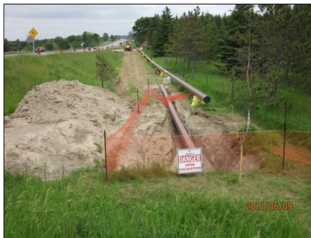
Figure 13 – The construction of a natural gas supply pipeline along Highway 9 has commenced. Nine kilometres (km) of the 16 km pipeline have been installed.
