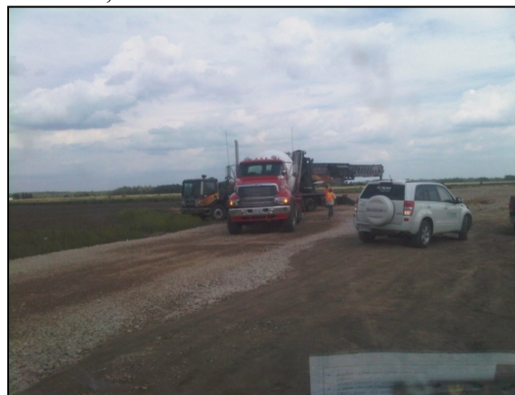
Figure 4 – The road use agreement with the Township of Melancthon has been executed and the road use agreement with the Township of Grey is being coordinated. Construction of access roads is also underway.
