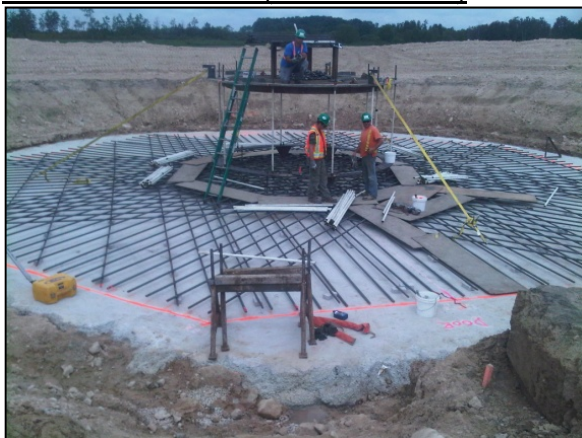
Figure 3 – Construction of foundations is underway.
