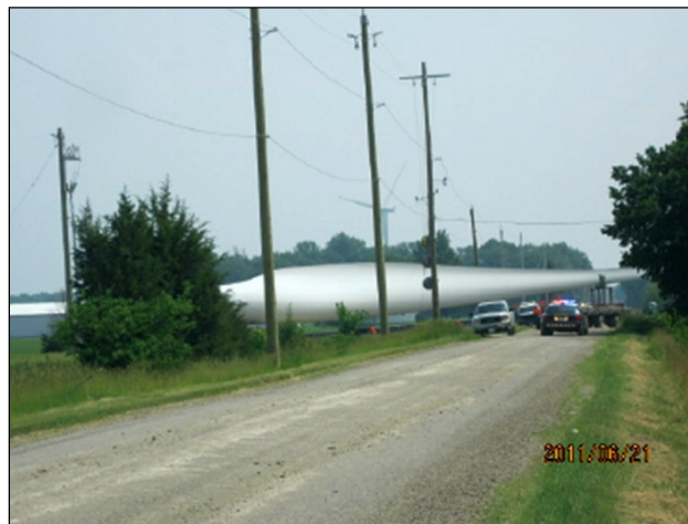
Figure 2 – One of the turbine blades being manoeuvred into the project site; in addition. Over 75 percent of foundations and access roads have been completed.
