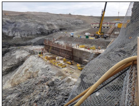
Figure 8 – The Smoky Falls rock stabilization work at the powerhouse excavation continues to progress, and two reinforced concrete pours at the intake have occurred.
