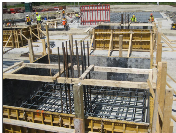
Figure 12 – Major equipment has been ordered and several powerhouse column footings are complete
