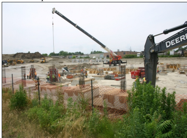
Figure 11 – Site construction activities have begun with site services and access road installed.
