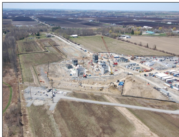
Figure 14 – Hydro One has installed the 230 kiloVolt (kV) interconnection support towers and tie-in loops. Exhaust stacks have been installed to full height, as have underground drainage and the fire water main. The structural steel for the control/warehouse building is in place and cladding is being installed. The turbine and generator are set and enclosures/auxiliaries are being installed.
