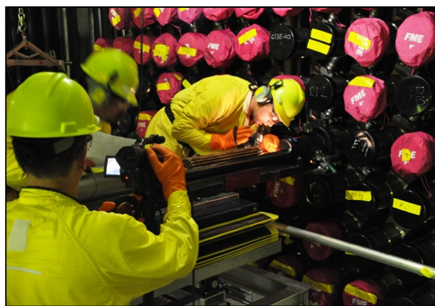
Figure 16 – The first fuel bundle was loaded into the refurbished Unit 2 reactor in June.
