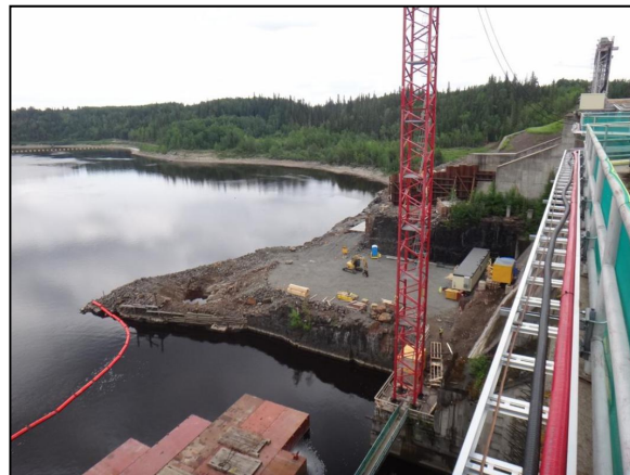
Figure 6 – Flexi-float pieces are being delivered to the site to facilitate in-water construction. The tower crane has been erected and commissioned.
