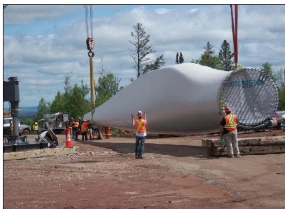
Figure 9 – The delivery of turbine components has begun at the project site. They are manufactured by Siemens.
