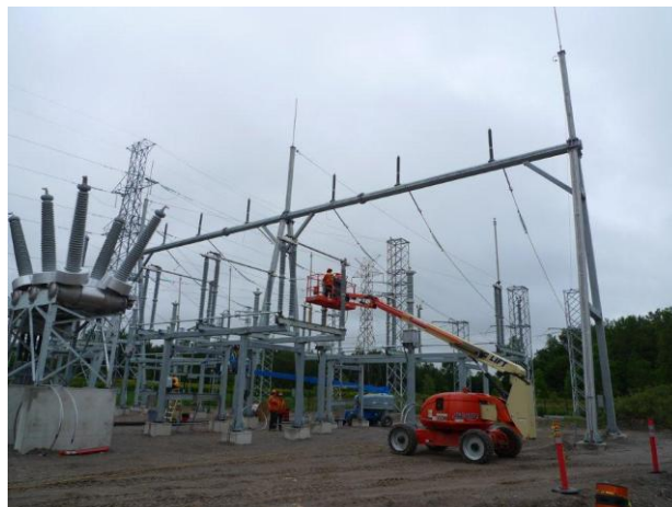
Figure 12 – Installation of conductors in the switch yard now completed and undergoing equipment testing.
