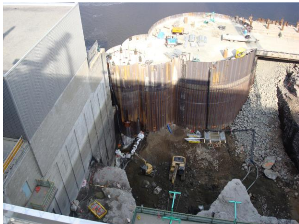
Figure 6 – The cofferdam was completed. Excavation of overburden, drilling and blasting operations have started in the de-watered area.
