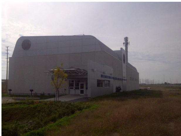
Figure 13 – Powerhouse building completed. Equipment installation inside the powerhouse in progress.
