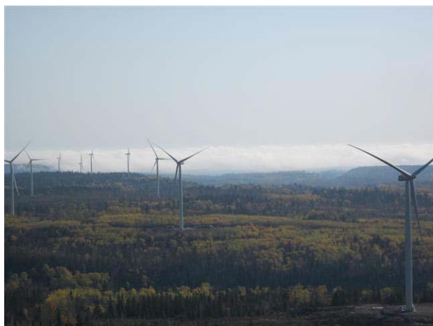
Figure 10 – Aerial view of the Greenwich wind turbine site. 43 Siemens turbines with a capacity of 2.3 MW each were fully assembled; 36 of these have been commissioned.
