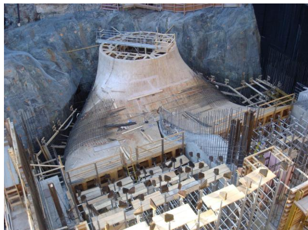
Figure 8 – The curved wood draft tube forms were in place and rebar was being installed in preparation for the draft tube pour. Other completed concrete pours include the penstock intake walls and invert, the central draft tube pier, and the east and west tailrace walls.
