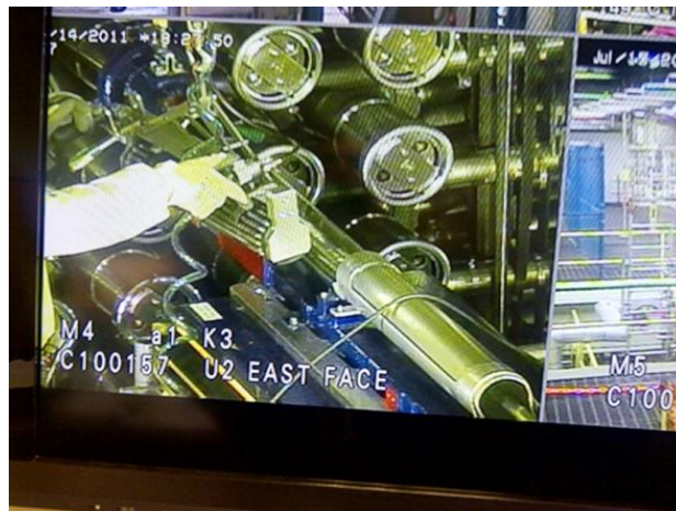
Figure 16 – The last of 5,760 new fuel bundles was loaded into the Unit 2 reactor in July. Fuel loading is a major milestone in the restart project.
