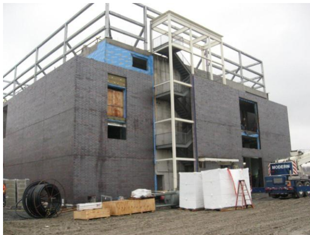
Figure 14 – Powerhouse construction is underway.
