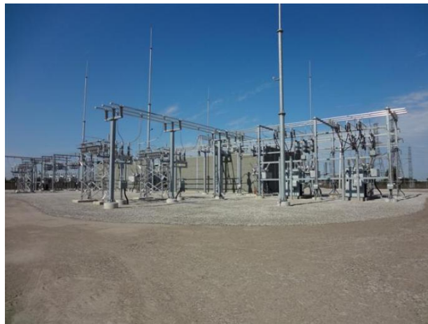
Figure 2 – Transmission system completed.
