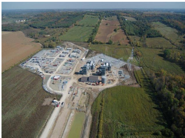
Figure 11 – Aerial view of the York Energy Centre. Major equipment installation near completion. Control/warehouse building structure erected and interior finishing was nearing completion.
