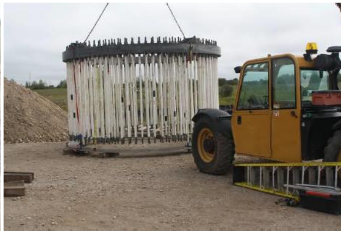
Figure 4 – Anchor bolt assembly ready for placement. Major equipment deliveries commenced. Construction has commenced at three of the five turbine sites.
