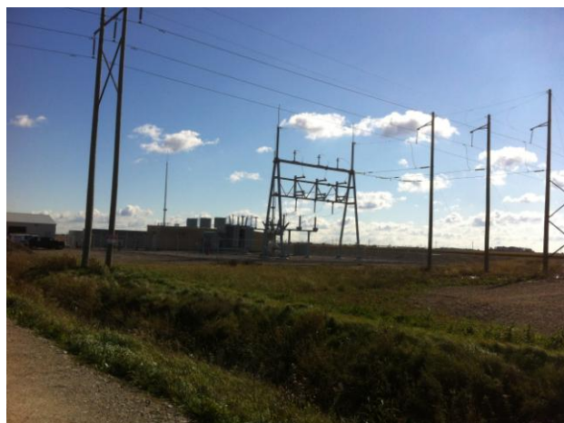
Figure 5 – Sub-station construction and transmission connections completed. All turbines pre-commissioned 100% complete. Construction for collector system 98% completed.
