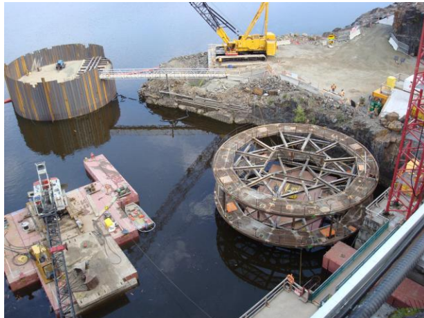
Figure 7 – One of the cofferdam cells is almost complete. Cleaning of the footprint for other cofferdam cells is in progress.
