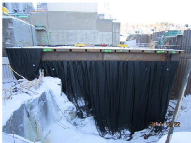
Figure 1: Drill and blast work progressed well in the powerhouse area. Concrete work started in mid-October and advanced quickly, the majority of the pours occurred at the intake. A winter shelter was erected for work during the winter months.
