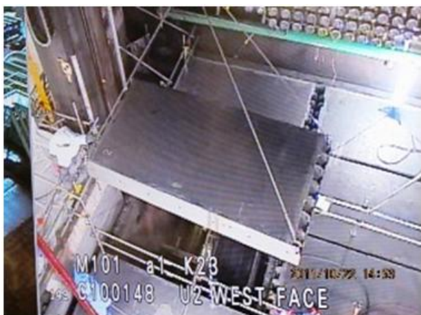
Figure 8: Bulkhead panel removed from unit 2 reactor vault.
