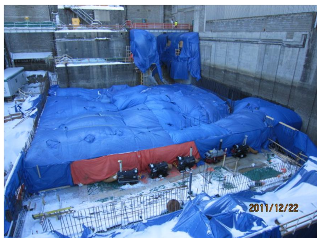
Figure 3: Concrete work continues to progress well in the powerhouse and intake areas. Preparatory work for the turbine and generator embedded parts and equipment installation is advancing.
