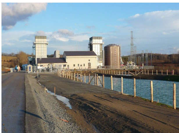
Figure 5: Unit #1 and #2 power train mechanical installation is nearing completion. Water storage tank installation is now complete.
