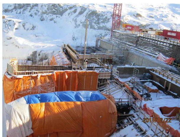
Figure 4: Concrete pours are progressing in the service bay, intake, and draft tube areas. Tailrace excavation continues, and a winter shelter was erected to allow concrete operations to continue during the winter months.
