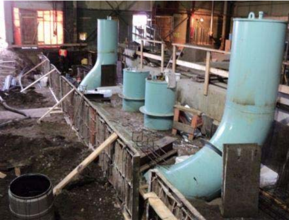
Photo 1 – Installation of condenser inlet and outlet piping in progress.
