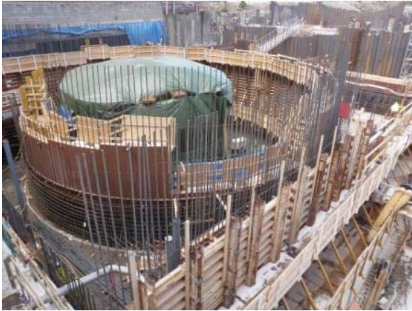
Photo 9 – Overview of progress around the powerhouse and intake areas, preparing for concrete pours.
