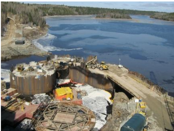
Photo 7 – Cofferdam cell #3 was installed and backfilled with sand.
