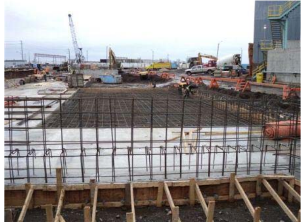
Photo 2 – Installation of rebar to support cooling tower base in progress.
