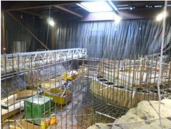
Photo 5 – Rebar installation continued during winter months inside a special winter shelter erected around the powerhouse footprint.
