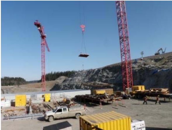
Photo 11 – View of the panel rigging and hoisting operations at the intake area.
