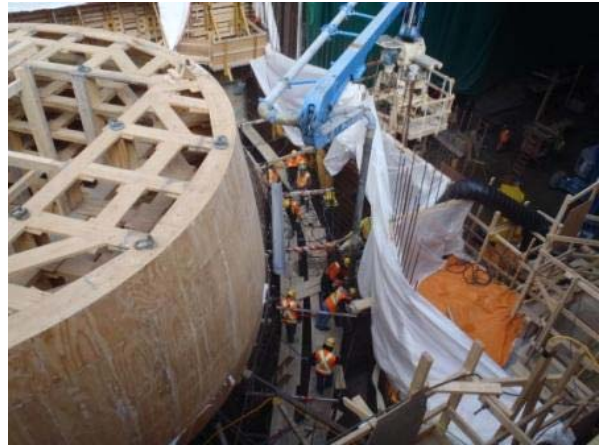
Photo 12 – Overview of the draft tube pour in progress.
