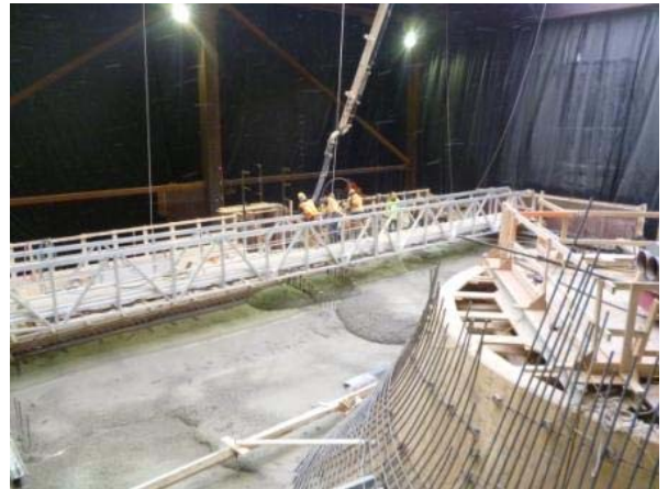
Photo 6 – Winter shelter erected around powerhouse area to allow concrete pours to continue in the winter months.
