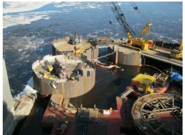
Photo 8 – Cleaning of the footprint for cofferdam #2 continued for steel shell installation.
