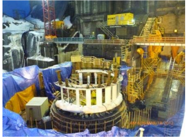
Photo 10 – Formwork and stay ring installed at the powerhouse.
