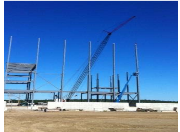
Photo 2 – The powerhouse structural steel erection in progress.
