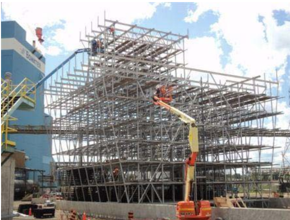
Photo 15 – The cooling tower under construction.
