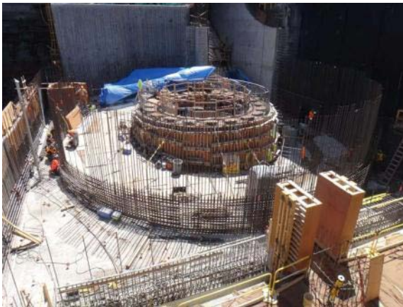
Photo 7 – A view of the concrete pour, with visible corrugated steel anchor guides.
