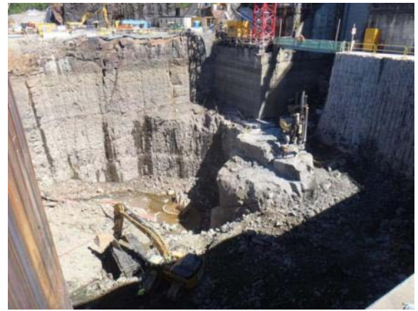
Photo 10 – Drilling and excavation in the Unit 3 footprint.
