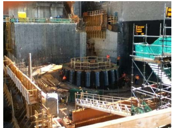
Photo 8 – Another view of the corrugated steel anchor guides embedded in concrete.
