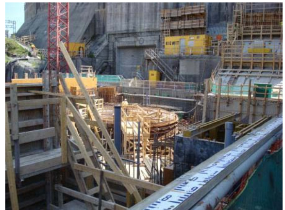
Photo 12 – A view of the concrete pour.
