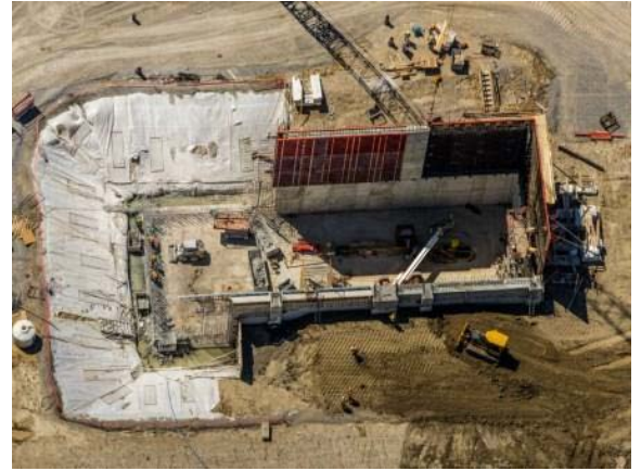
Photo 6 – An aerial view of the refuse pit under construction.
