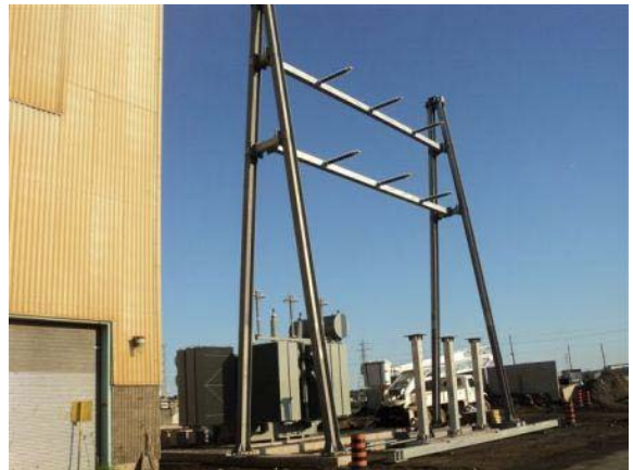
Photo 16 – The TG6 substation in progress.
