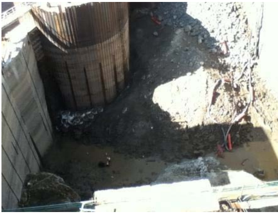
Photo 9 – A view of the dewatered lagoon.
