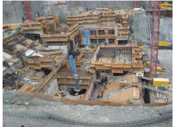
Photo 14 – A view from the east bank of the Mattagami River.
