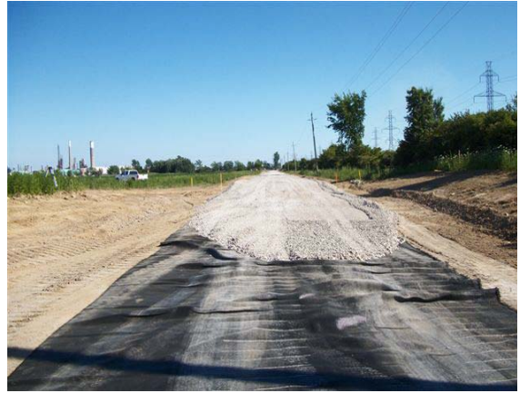
Photo 10 – A view of an entrance road under construction.
