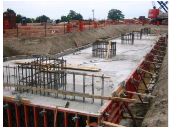
Photo 4 – Turbine generator pedestal and foundations were completed.
