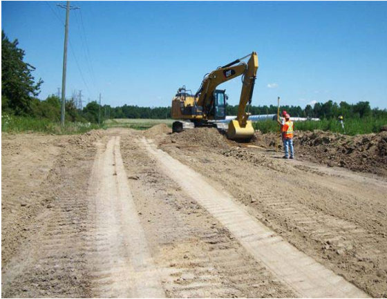
Photo 9 – Construction of an entrance road to the point of interconnection was started.
