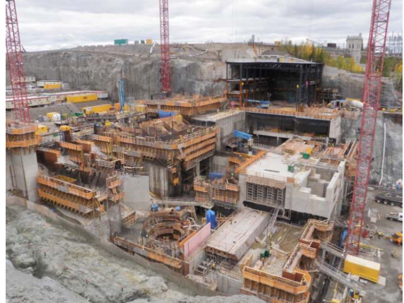
Photo 8 – Concrete pours continued to progress in the service bay, intake and draft tube areas.
