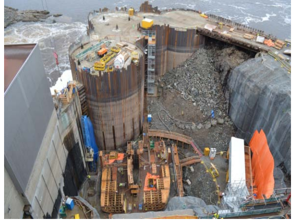
Photo 6 – Concrete work was proceeding in the intake and powerhouse areas.
