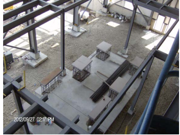
Photo 2 – The turbine foundations located inside the generating facility building were completed.
