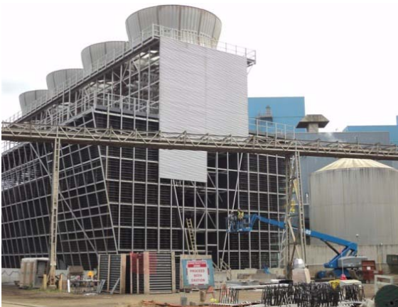
Photo 11 – Cooling tower structure was 95 percent complete.
