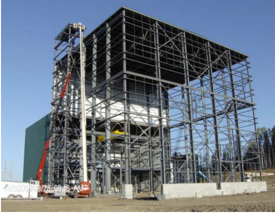
Photo 1 – Generating facility building was in progress with bridge crane being installed. The building, which has an overall dimension of approximately 60 x 24 meters, will house most of the plant equipment.
