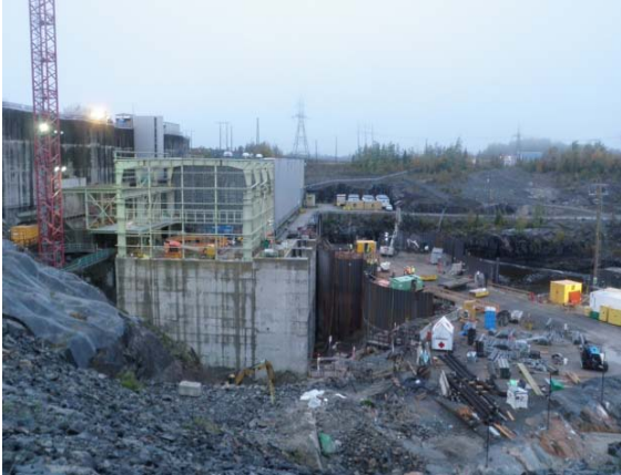
Photo 7 – The draft tube gates were installed and the area behind the cofferdam was watered up.
