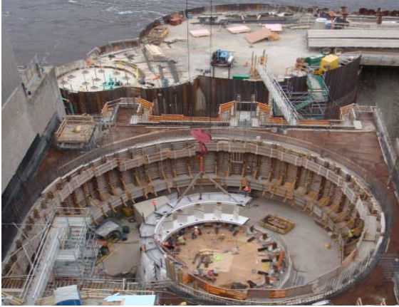
Photo 5 – The installation of turbine embedded parts was nearing completion.
