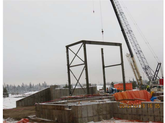
Photo 2 – Structural steel erection was under way
