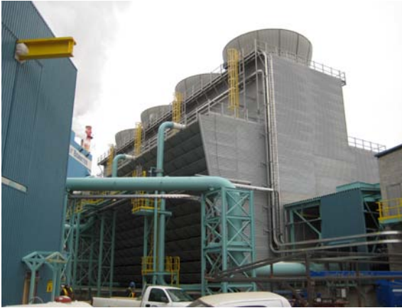
Photo 11 – Erection of cooling tower was nearing completion
