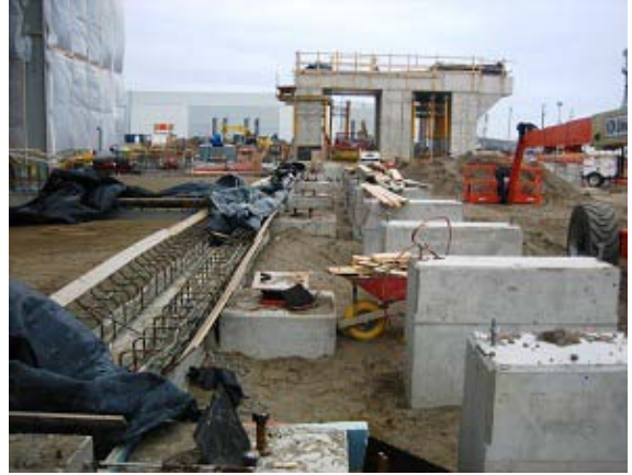
Photo 6 – Vibrating conveyor pedestals and boiler slab preparation were in progress
