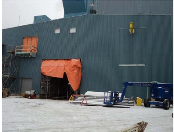
Photo 12 – Construction of electrical annex was in progress
