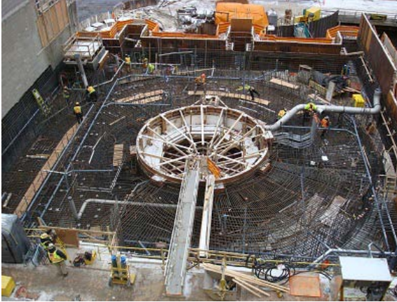
Photo 7 – Concrete was in progress, installation of major turbine embedded parts was completed
