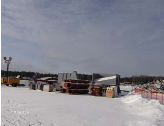
Photo 3 – Boiler parts were delivered
