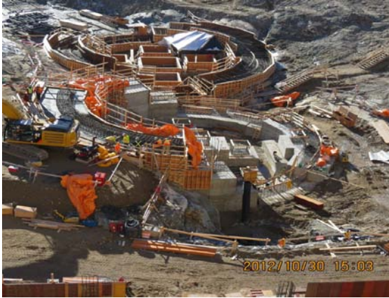
Photo 1 – Foundation concrete forming and pouring were under way
