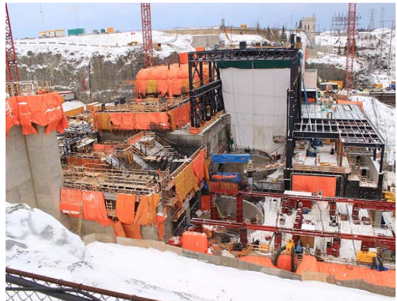
Photo 10 – Concrete work and powerhouse steel frame erection continued to progress well. Tarps had been installed and prepared for winter construction
