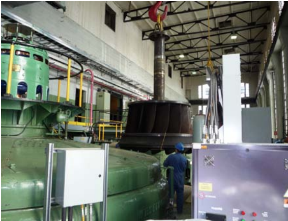
Photo 13 – Old turbine runner was being removed
