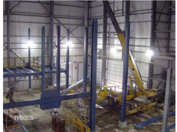
Photo 4 – Boiler support steel erection was under way
