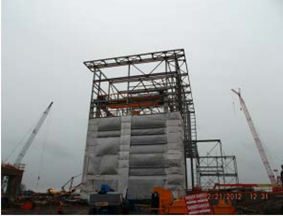
Photo 5 – Refuse building and tipping building construction were in progress
