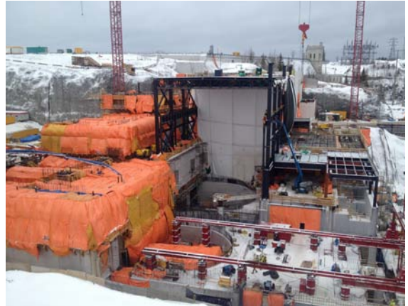
Photo 10 – The superstructure over units 1 and 2 was enclosed with tarps and heated for winter construction
