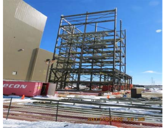
Photo 2 – Structural steel erection was progressing
