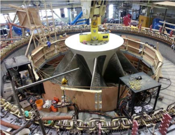
Photo 9 – Runner for the additional unit of 67 MW was lowered into pit
