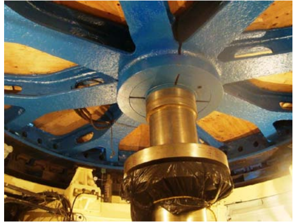
Photo 16 – Generator rotor turbine shaft was coupled
