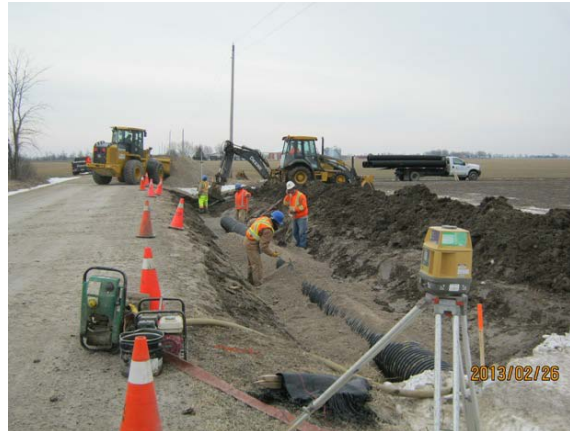
Photo 14 – Drain pipe was being installed and backfilled as part of the access road construction
