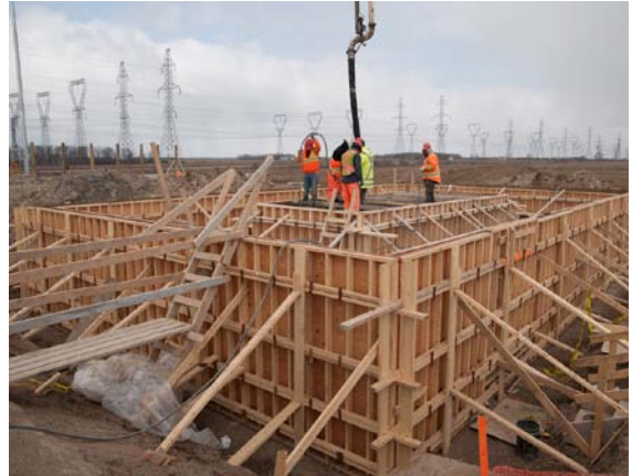
Photo 12 – The main transformer foundation was under way
