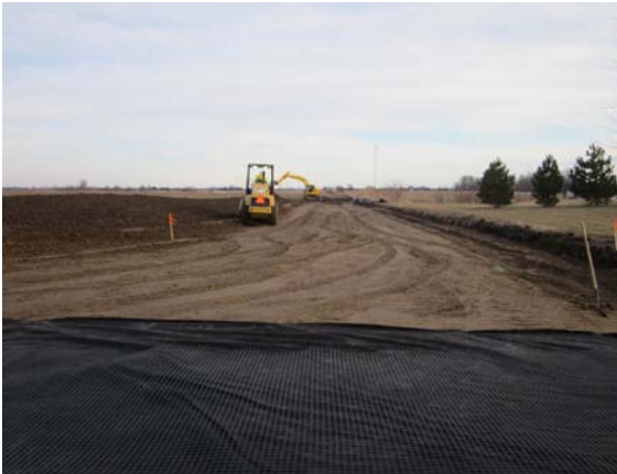
Photo 13 – Access road was being formed, levelled and prepared for laying geogrid mat. A geogrid mat is a geosynthetic material used to reinforce soil in the sub-base of road work
