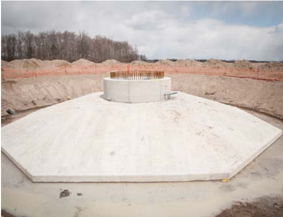
Photo 11 – One of the 58 turbine foundations was completed
