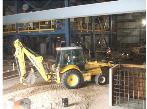
Photo 4 – Turbine hall floor leveling was under way
