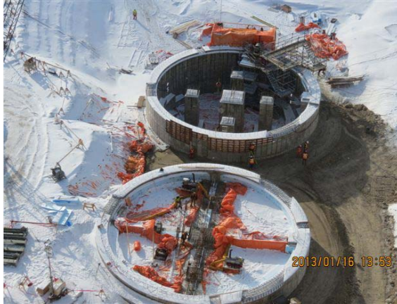
Photo 1 – Foundation concrete forming and pouring were progressing
