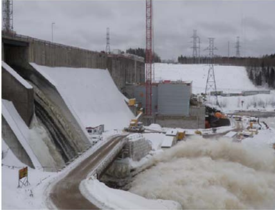
Photo 7 – Unit 3 with a capacity of 78 MW was enclosed and jointed to the existing power house
