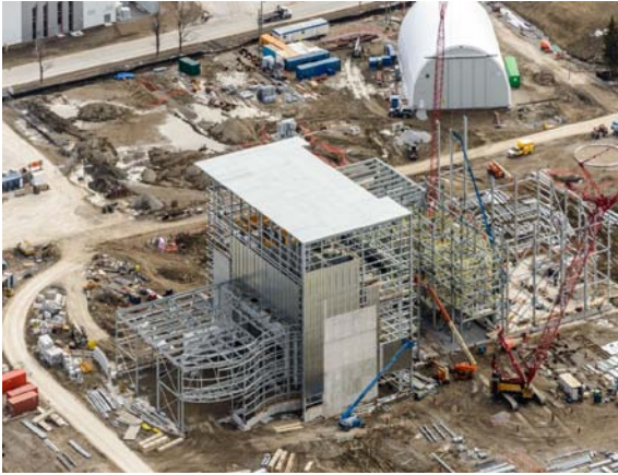
Photo 5 – An aerial view of Durham York Energy Centre construction site
