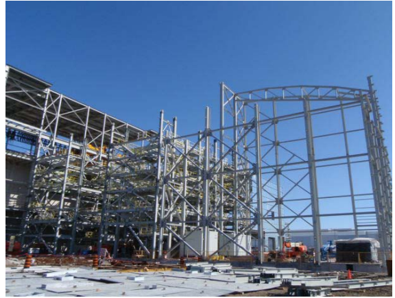
Photo 6 – Boiler and air pollution control steel were erected
