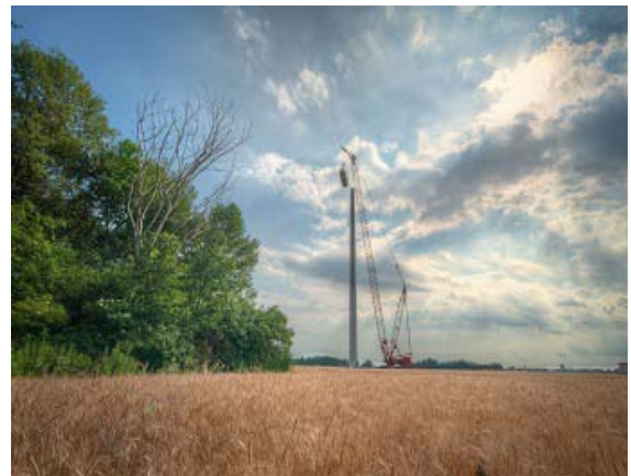
Photo 14 – The nacelle lift was in progress
