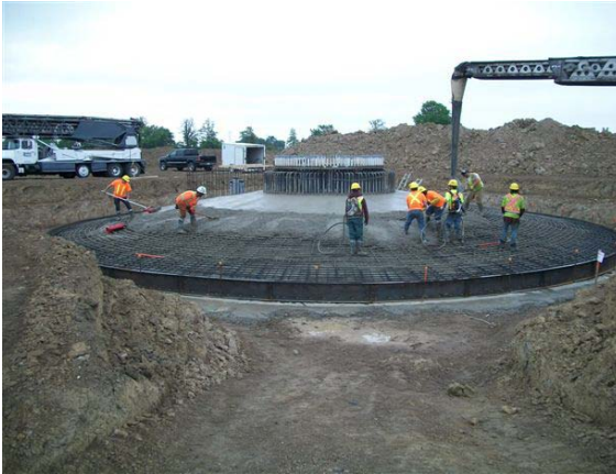
Photo 15 – One of the wind turbine foundation pours was in progress
