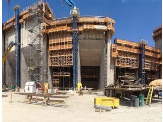
Photo 10 – Concrete pouring continues to progress in the service bay, intake and powerhouse areas
