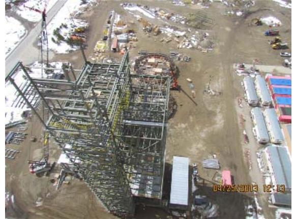
Photo 2 – Transfer tower structural steel erection was completed
