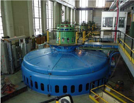
Photo 19 – After runner upgrade, generator 4 was nearing final stages of re-assembly
