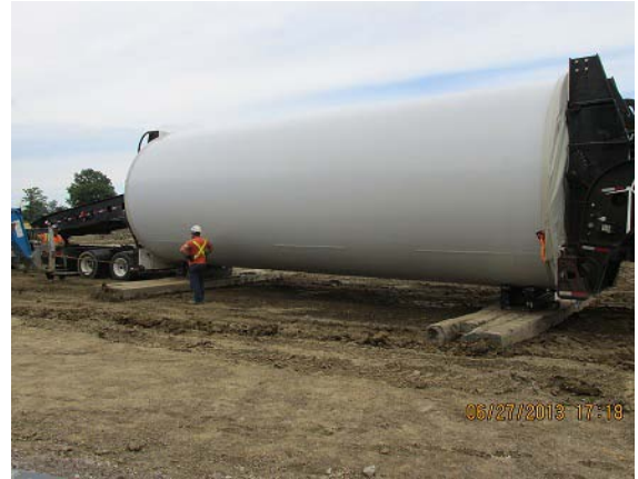
Photo 16 – The first wind turbine generator base was delivered on site
