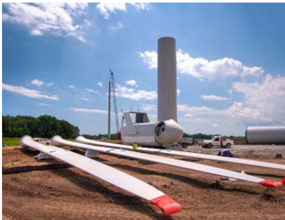
Photo 13 – The wind turbine component preparation for assembly was in progress
