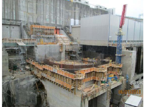
Photo 8 – Concrete work resumed in unit 3
