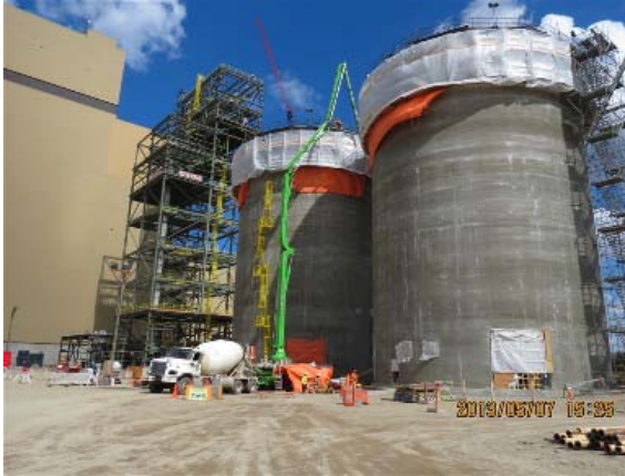
Photo 1 – Silo slip forming was completed
