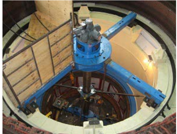
Photo 20 – The generator 5 on-site machining was in progress
