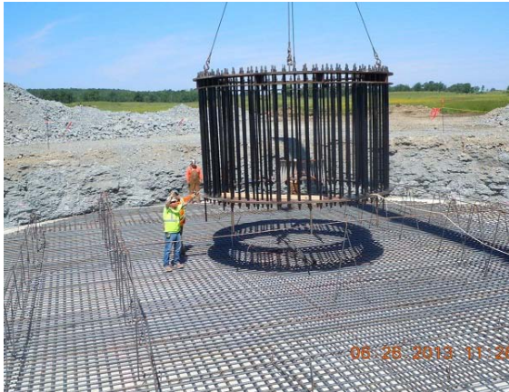
Photo 11 – Turbine foundation rebar and tower anchor bolts installation was in progress
