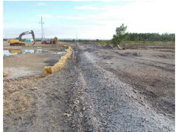
Photo 12 – Cable trenching for submarine cable was completed
