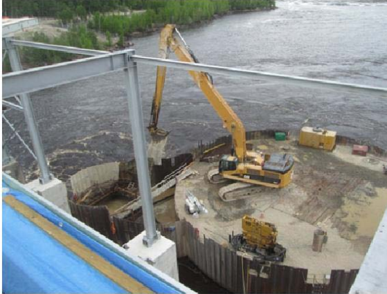
Photo 7 – Cofferdam removal was in progress
