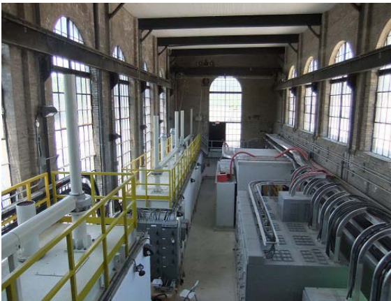
Photo 17 – New powerhouse interior was completed
