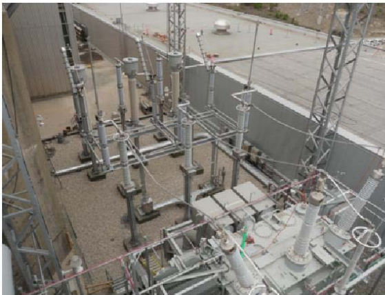
Photo 9 – Switchyard of unit 3 was completed
