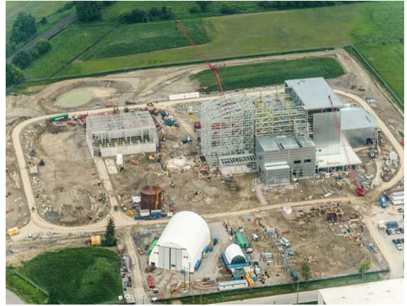
Photo 6 – Building liner panels and roofing in the tipping building, refuse building and turbine generator building were completed
