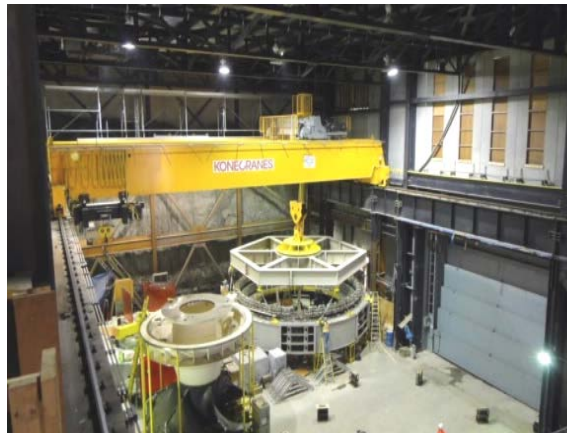
Photo 10 – Unit 1 stator lift
