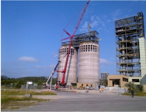
Photo 1 – Silo internals installed and roof cement poured
