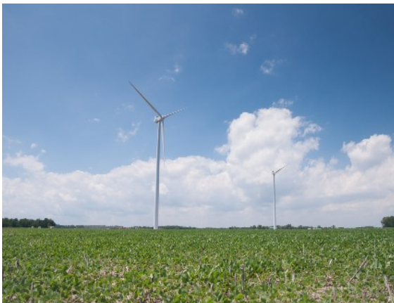
Photo 13 – Two of the 30 turbines that achieved mechanical completion
