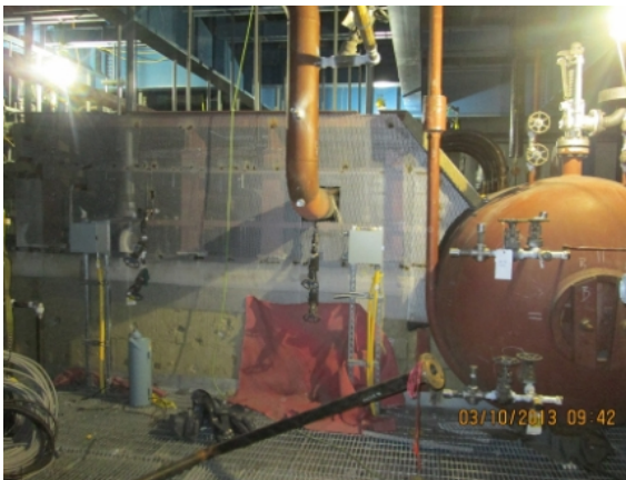
Photo 3 – Cladding of boiler penthouse installed
