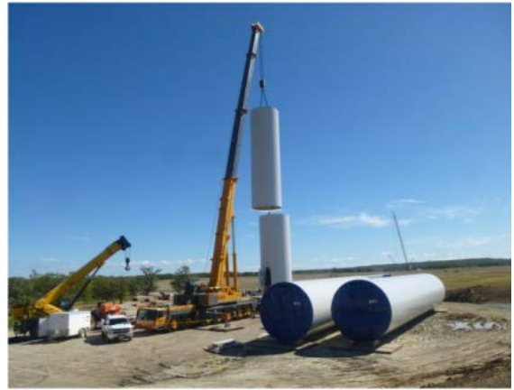
Photo 12 – Stacking tower sections by installing lower-mid section onto tower base
