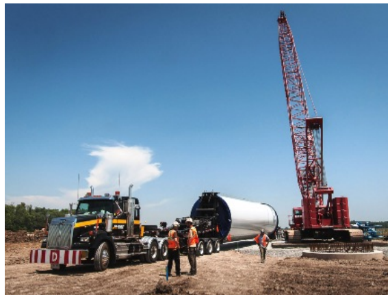
Photo 14 – Construction continuing on the remainder of turbine bases
