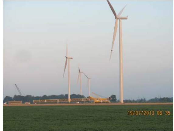
Photo 16 – Several of the turbines that achieved mechanical completion
