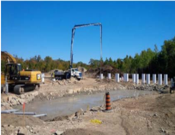
Photo 11 – Concrete pouring for control building support piers
