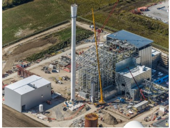
Photo 6 – Stack has been erected
