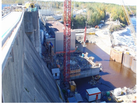
Photo 8 – Work area behind cofferdam watered up
