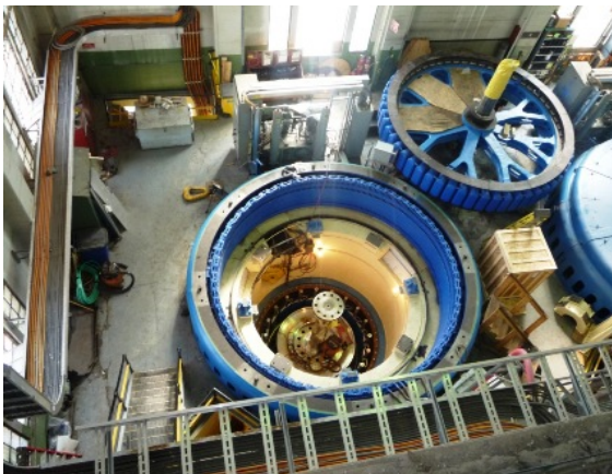
Photo 17 – Installation of the new runner for Generator 5
