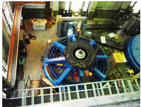
Photo 18 – Reassembly of the Generator 5 rotor, stator and exciter
