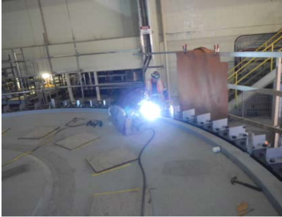
Photo 7 – Rotor welding
