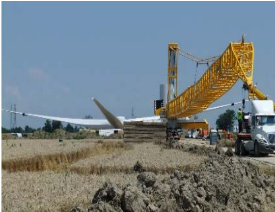
Photo 15 – Main crane assembly in preparation to lift turbine blades
