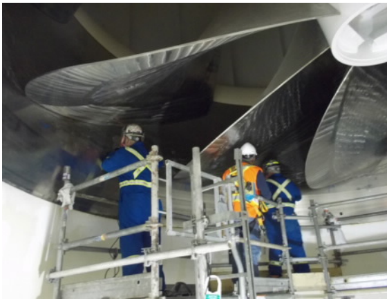
Photo 9 – Discharge ring inspection
