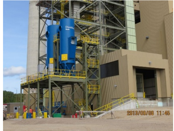
Photo 2 – Transfer tower construction continued
