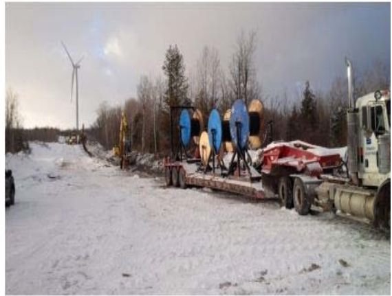
Photo 20 – Installing the collection system cables
