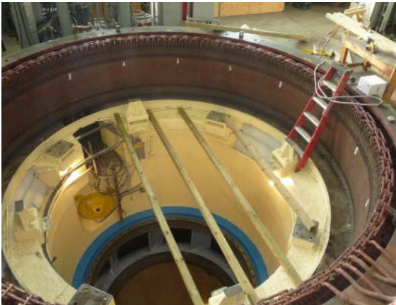
Photo 25 – Generator 3 turbine pit work completed
