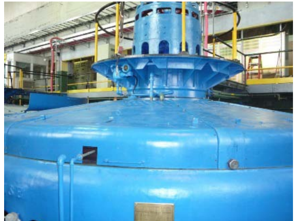
Photo 26 – Generator 5 completed and awaiting commissioning
