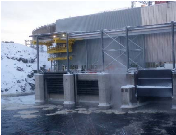
Photo 17 – Plant infrastructure near completion
