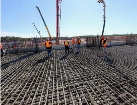
Photo 13 – Pouring concrete for the base of the heat-recovery steam generator
