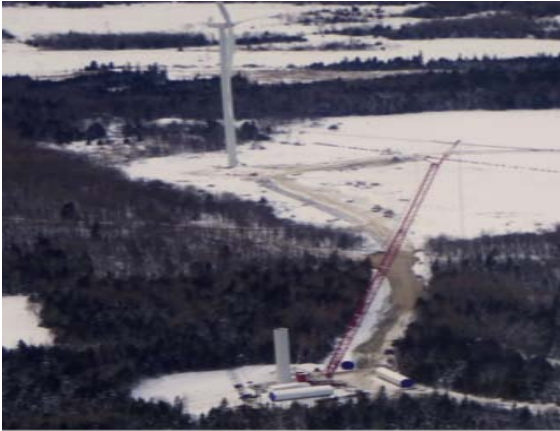
Photo 19 – Installing a wind turbine stack
