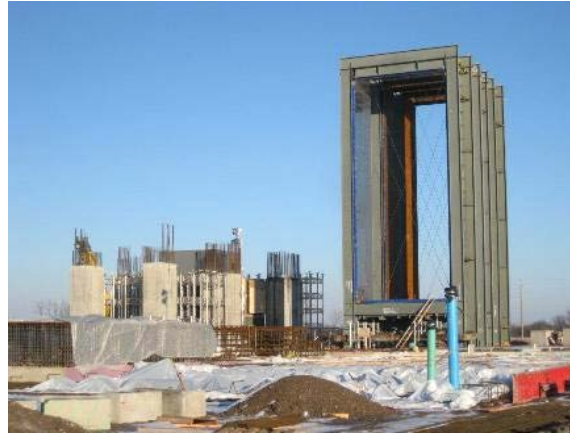
Photo 14 – Building the casing and stack assembly for the heat-recovery steam generator
