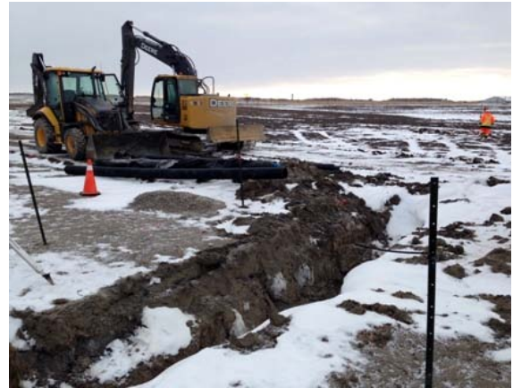
Photo 2 – Site preparation work: laying drain pipes
