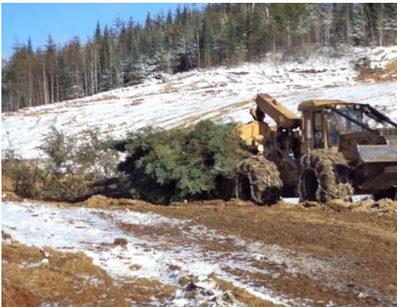
Photo 11 – Site preparation work: clearing and stacking trees
