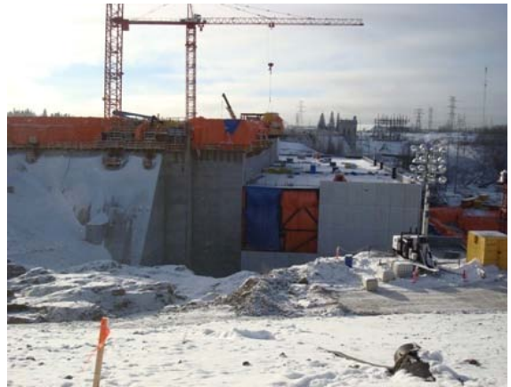
Photo 18 – Building the retaining walls of the dam
