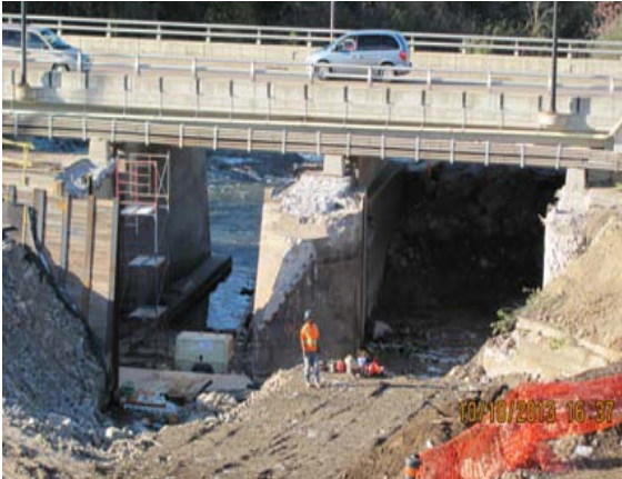
Photo 23 – Demolishing the deck of the upper dam
