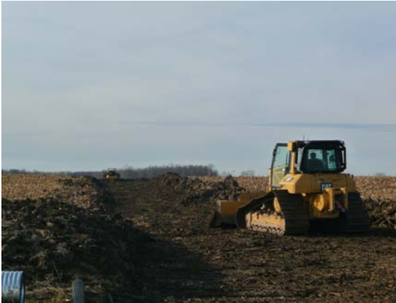
Photo 5 – Site preparation work: cutting an access road
