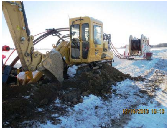
Photo 8 – Installing the collection system cables
