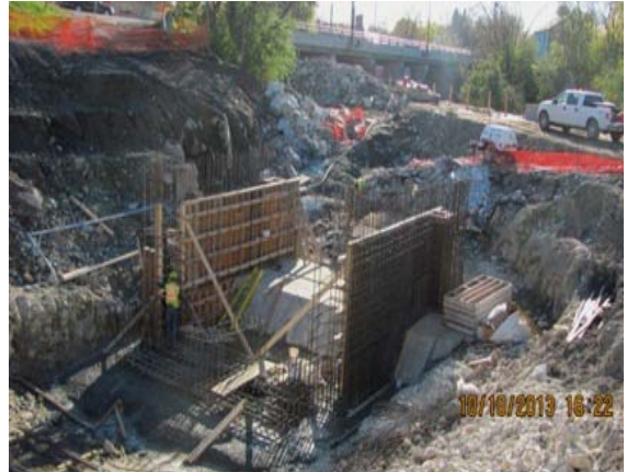
Photo 24 – Building the foundation of the headworks
