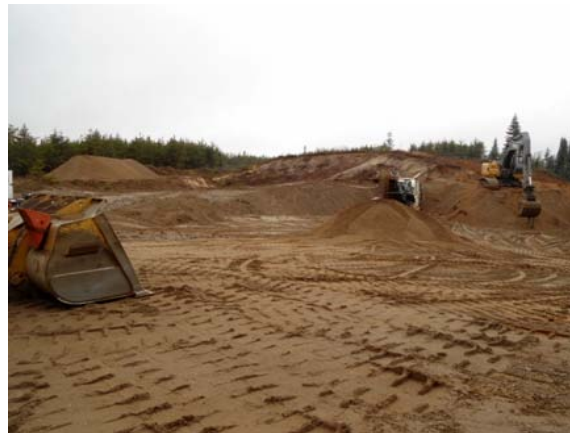
Photo 12 – Building the sand-crushing borrow pit
