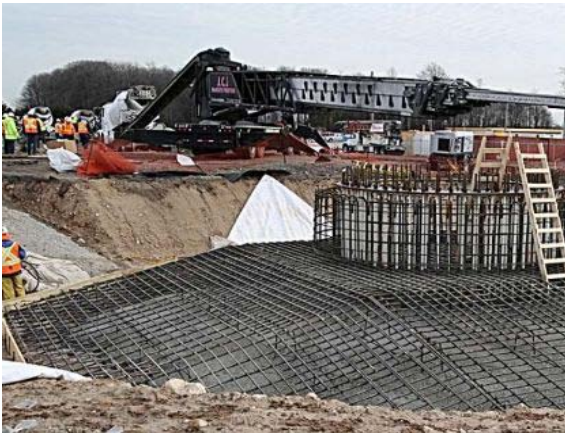
Photo 7 – Building the foundation of a wind turbine stack
