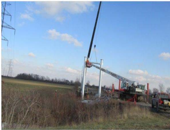
Photo 21 – Assembling the components of a turbine stack
