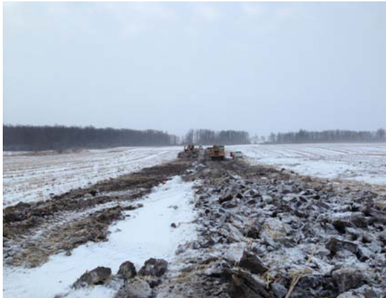
Photo 1 – Site preparation work: stripping a roadway
