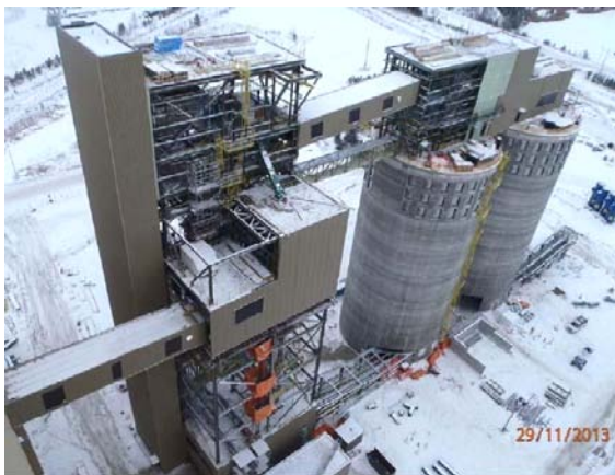
Photo 3 – Installing cladding on the silo conveyor
