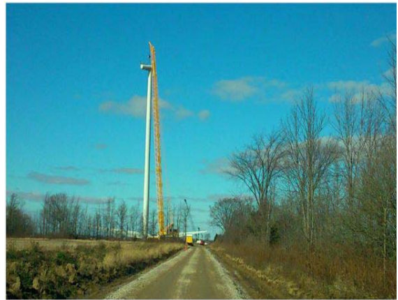
Photo 22 – Erecting a wind turbine stack
