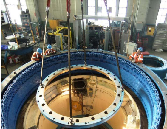
Photo 25 – Lowering the bottom ring of Generator 3 into position
