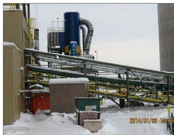
Photo 4 – View of conveyor at the silo base
