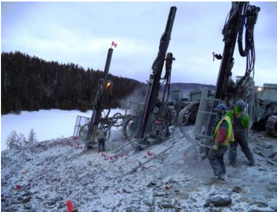
Photo 11 – Drilling shear lines for the diversion channel
