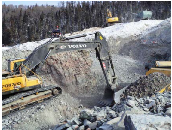
Photo 12 – Removing rocks in the spillway channel
