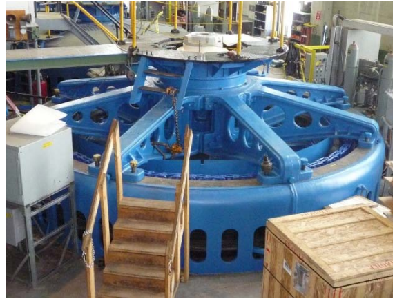
Photo 26 – Reassembling Generator 3
