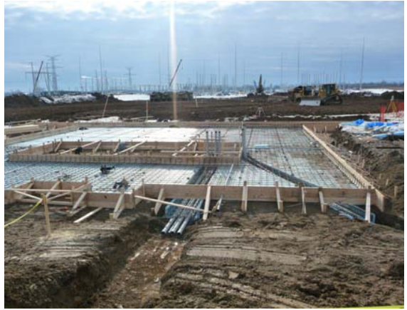
Photo 6 – Erecting the containment for a generator step-up transformer
