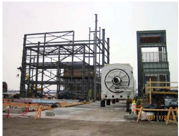
Photo 16 – Building the casing and stack assembly for the heat-recovery steam generator
