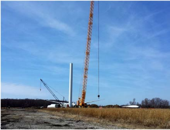
Photo 13 – Assembling the components of a turbine stack
