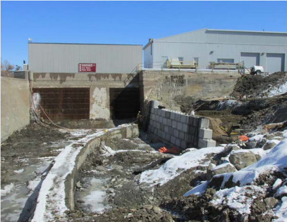
Photo 23 – Constructing the inner canal wall
