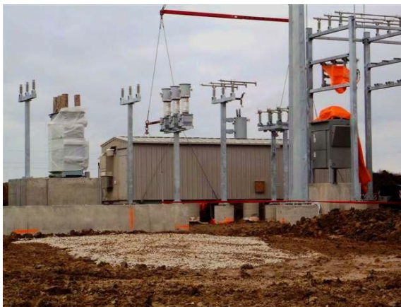
Photo 1 – Substation work: setting the control house
