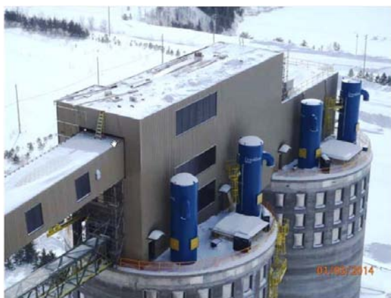
Photo 3 – Installing cladding on the silo conveyor
