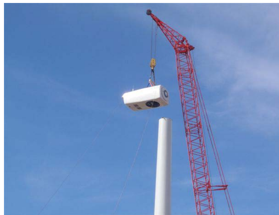
Photo 2 – Turbine work: erecting Nacelle T2 -3
