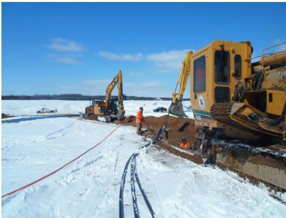
Photo 7 – Installing the collection system cables
