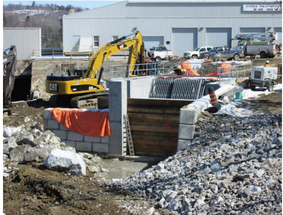
Photo 24 – Constructing the headworks of the dam
