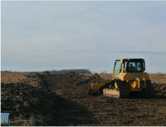
Photo 5 – Site preparation work: cutting an access road
