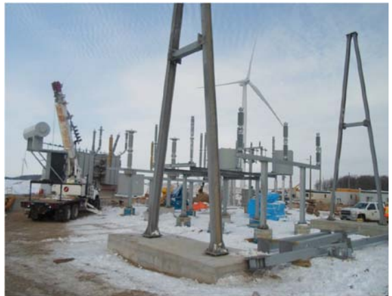
Photo 8 – Constructing the substation
