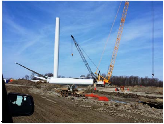
Photo 14 – Erecting a wind turbine stack
