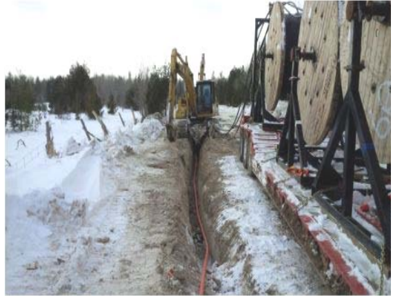
Photo 22 – Installing fiber-optic collector cable and conduit
