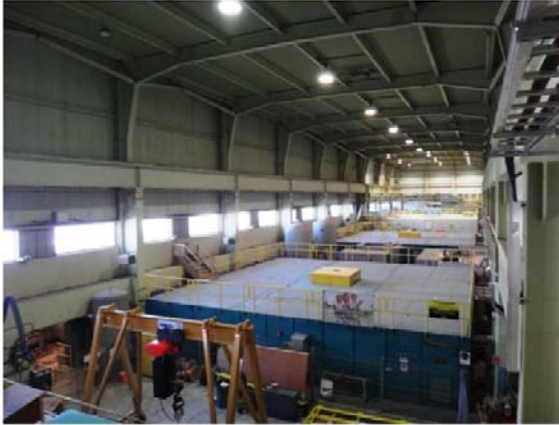
Photo 17 – Interior view of the turbine hall
