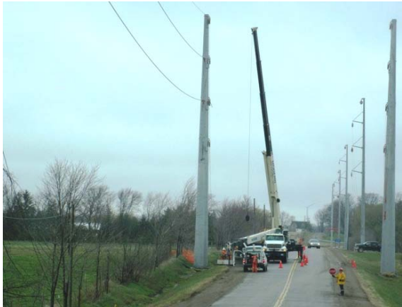
Photo 1 – Constructing the Kerwood Road transmission line
