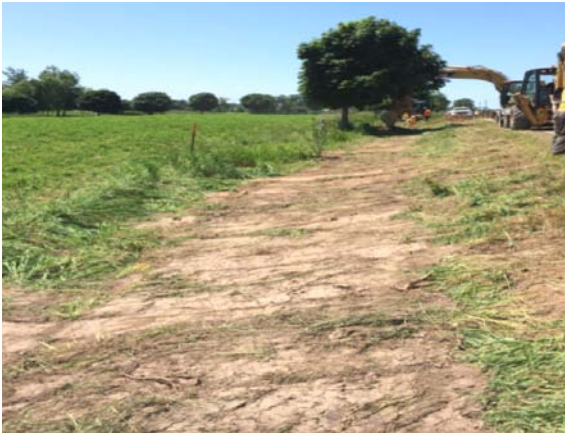
Photo 19 – Installing conduits along Hawkins Road
