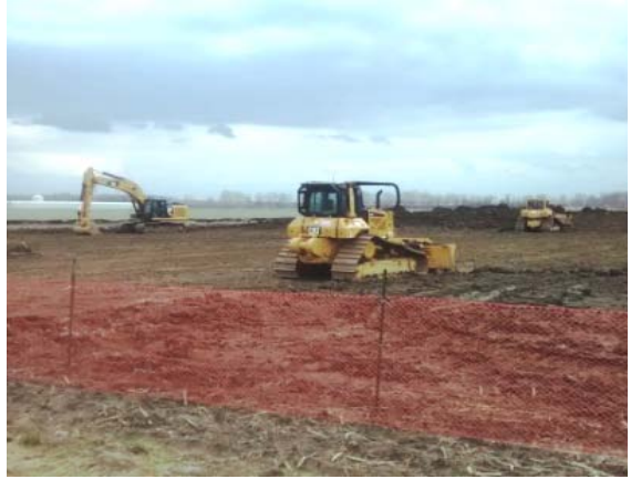
Photo 22 – Site work: preparation
