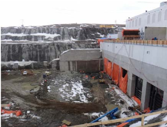
Photo 25 – View of the tailrace
