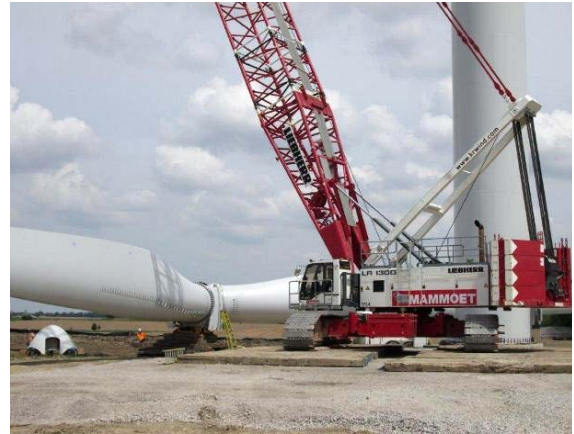
Photo 2 – Turbine work: constructing wind turbine WTG 25
