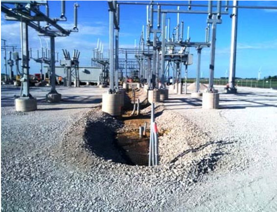
Photo 5 – Installing cables in the substation
