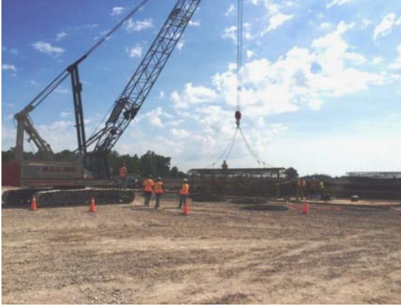
Photo 21 – Construction of the caissons
