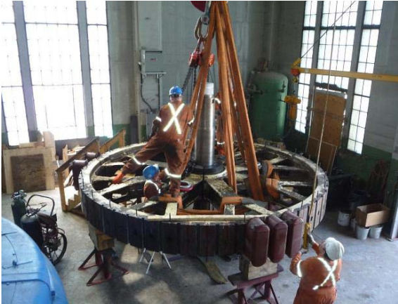
Photo 30 – Disassembling the rotor of Generator 2
