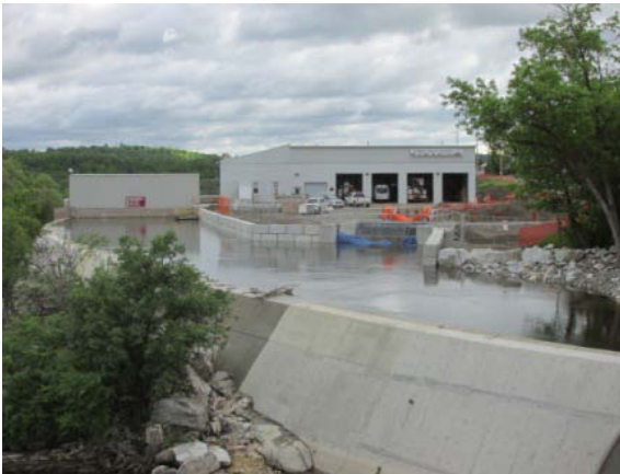
Photo 28 – Completed canal and headworks
