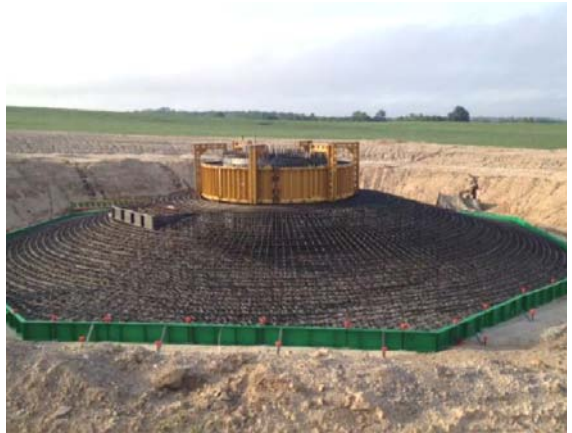
Photo 20 – Reinforcement bars forming the base of a turbine stack
