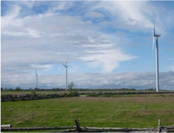
Photo 26 – The wind farm now in commercial operation
