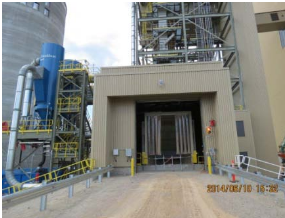
Photo 3 – Front view of the silo conveyor
