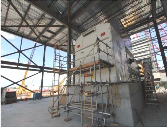
Photo 17 – Setting the main generator in place
