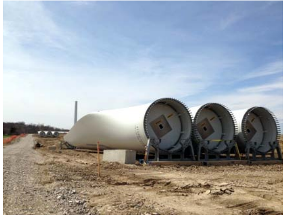
Photo 6 – Turbine stacks laid out prior to installation
