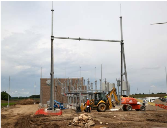
Photo 7 – Constructing the substation
