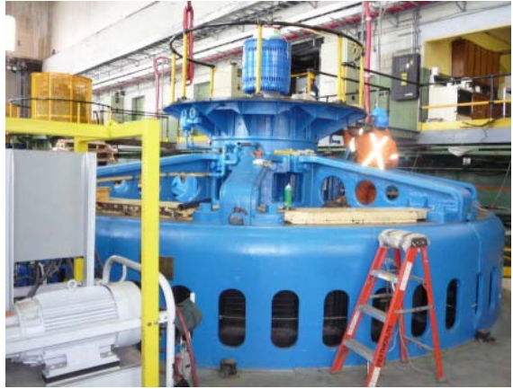
Photo 31 – Work on Generator 3 nearing completion
