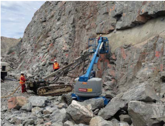
Photo 11 – Air track drill work on wall of diversion channel
