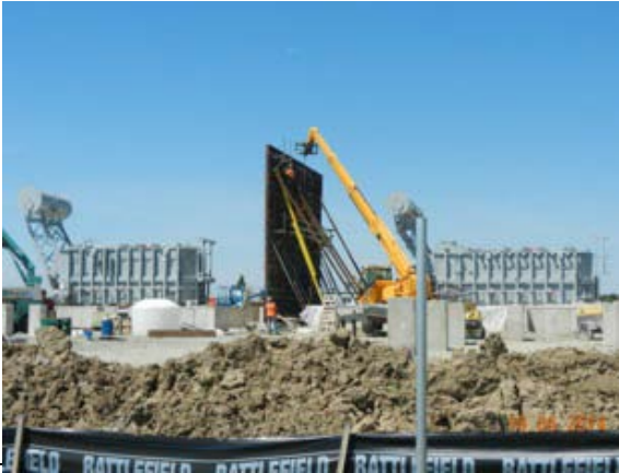
Photo 13 – Preparing the site for construction
