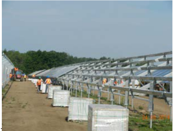
Photo 14 – Installing the racks used to house solar panels
