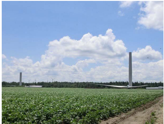
Photo 8 – Turbine blades laid in place prior to installation
