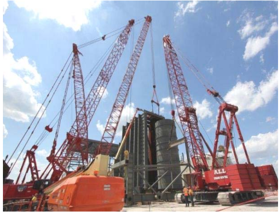
Photo 18 – Building the casing and stack assembly for the heat-recovery steam generator
