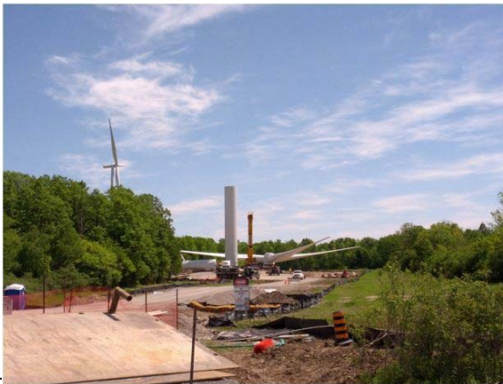
Photo 15 – Assembling the components of a turbine stack
