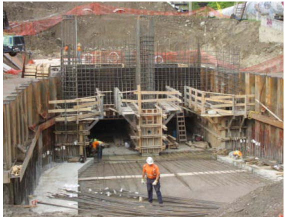
Photo 29 – Constructing powerhouse foundation and headworks
