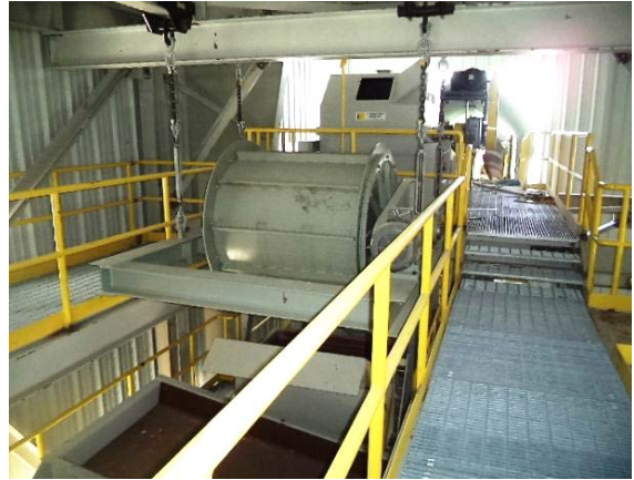
Photo 10 – Internal view: rotary drum magnet
