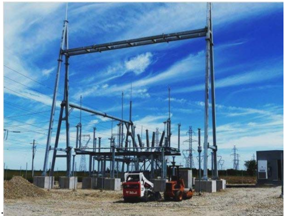
Photo 16 – Construction work at the switchyard
