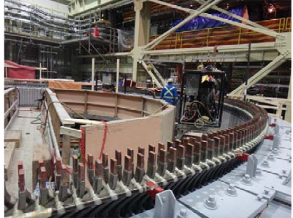
Photo 24 – Stator winding in progress
