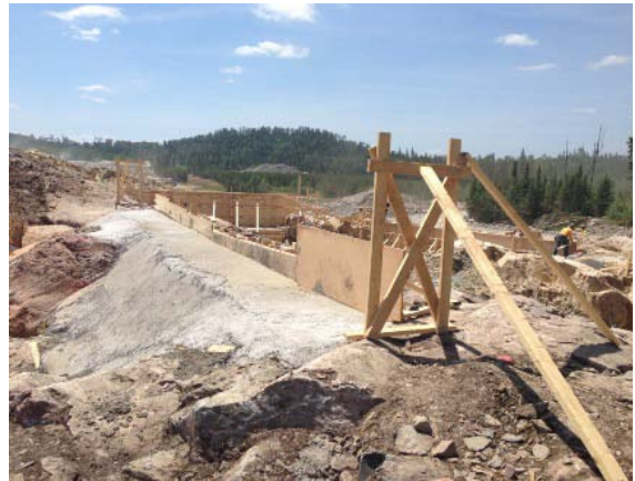
Photo 12 – Constructing the sedimentation tank
