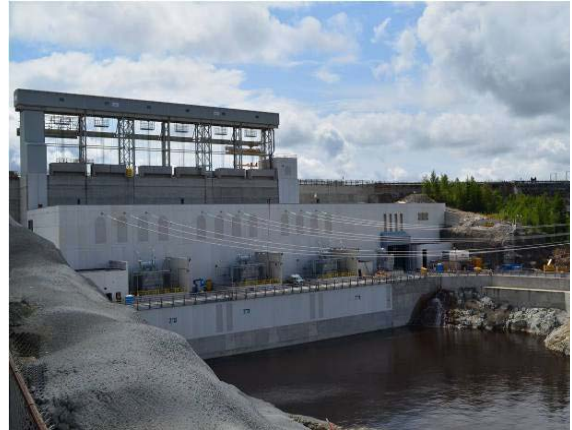
Photo 18 – View of the powerhouse and tailrace
