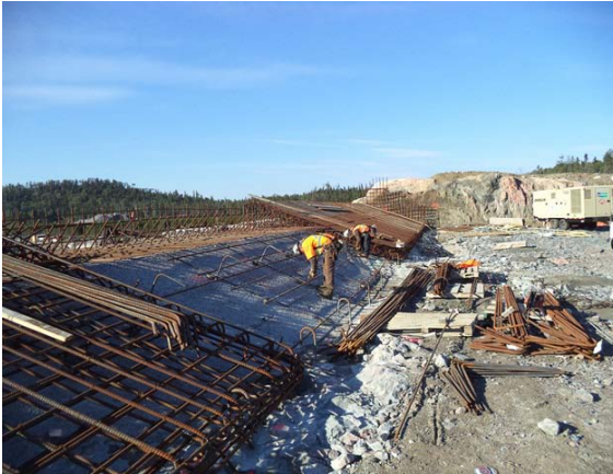
Photo 5 – Installing reinforcing bars in the overflow spillway area
