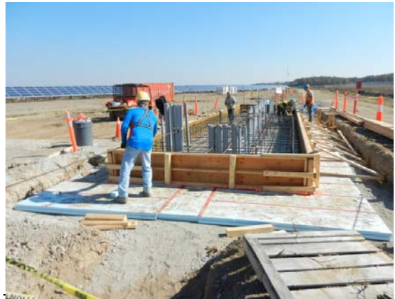
Photo 8 – Constructing infrastructure for the solar farm
