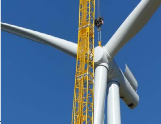
Photo 9 – Installing turbine blades on a wind stack
