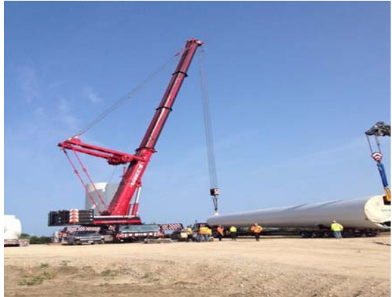
Photo 14 – Offloading the T200 turbine stack
