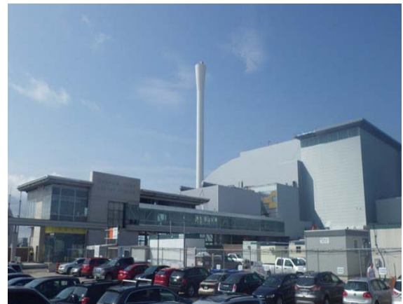
Photo 4 – Southwest view of the nearly completed facility
