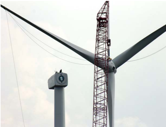
Photo 15 – Installing turbine blades on a wind stack
