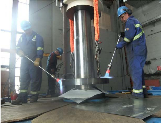
Photo 21 – Heating top rotor keeper ring of Generator 2
