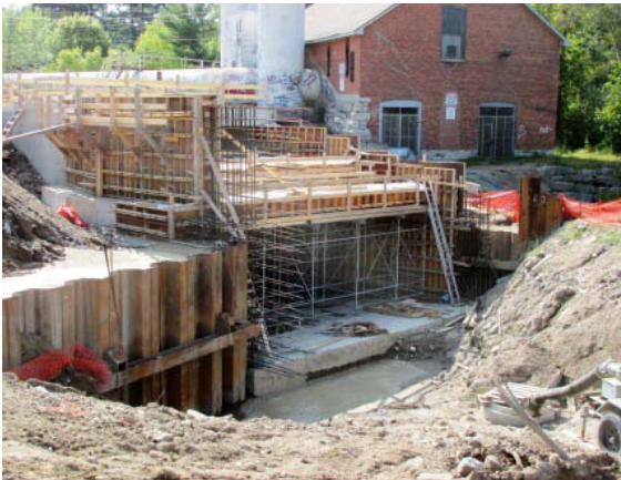
Photo 19 – Constructing the powerhouse tailrace
