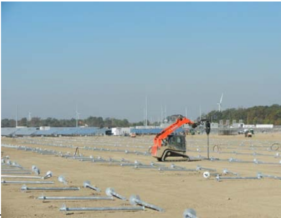
Photo 7 – Laying out framing for solar panel racks
