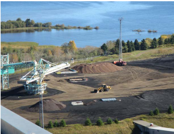
Photo 23 – Aerial view of advanced biomass processing
