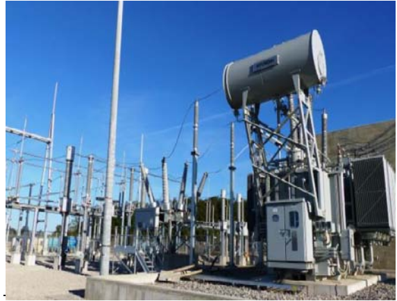
Photo 10 – Construction work at the switchyard
