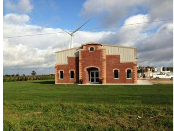
Photo 2 – View of the operations and maintenance building
