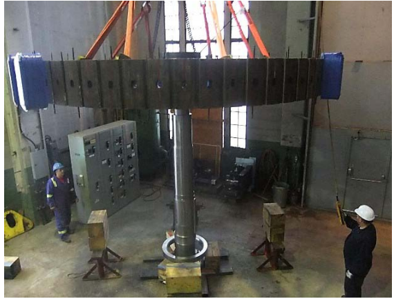
Photo 22 – Mounting the rotor on the shaft of Generator 2
