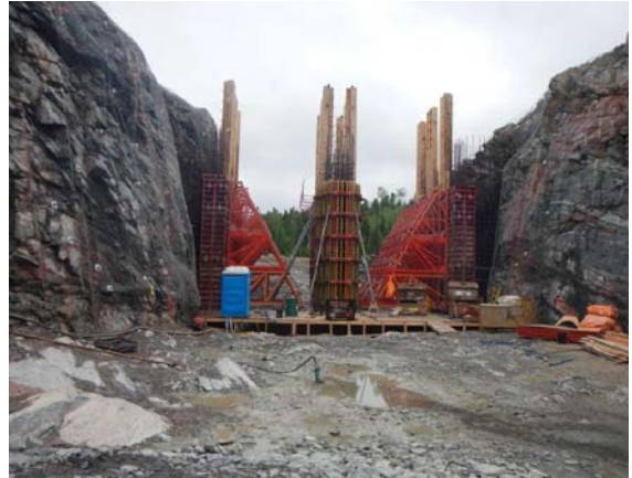
Photo 6 – Constructing the upper site low-level spillway
