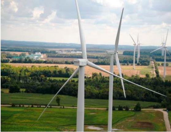
Photo 1 – View of several installed wind turbines
