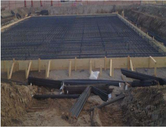
Photo 13 – Constructing a transformer foundation slab
