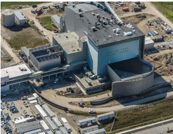
Photo 3 – Aerial view of the nearly completed facility
