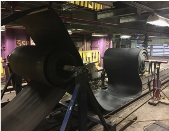
Photo 21 – Conveyor belt replacement
