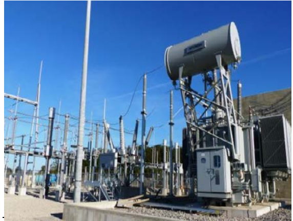
Photo 10 – Construction work at the switchyard
