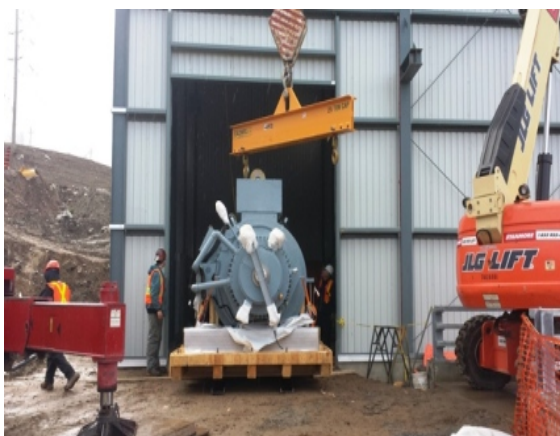
Photo 18 – Installing the generators
