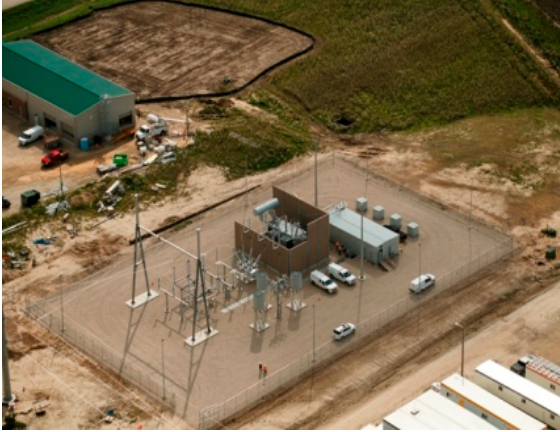
Photo 1 – View of the completed facility substation
