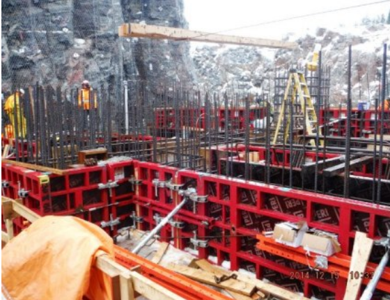
Photo 5 – Installing reinforcing bars in the soffit
