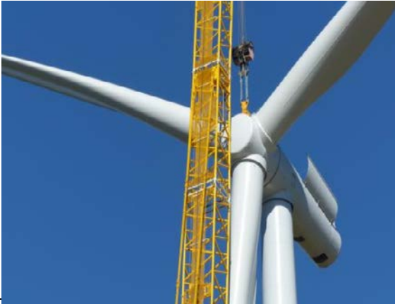
Photo 9 – Installing turbine blades on a wind stack
