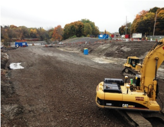
Photo 15 – Excavating the site for the powerhouse
