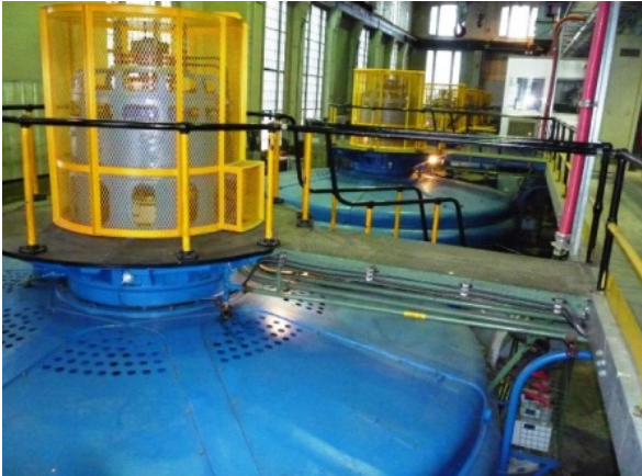
Photo 20 – View of Units 1-5 completed and installed
