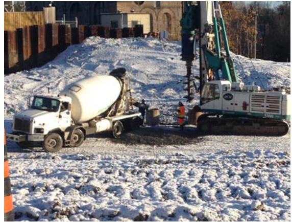
Photo 16 – Caisson installation
