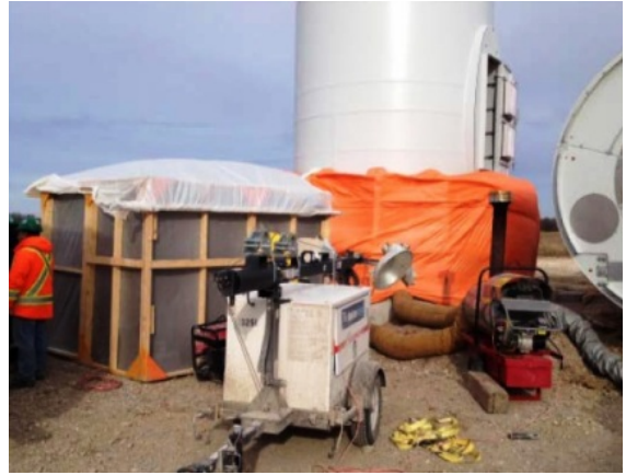
Photo 14 – Heating and hoarding for grout at T308
