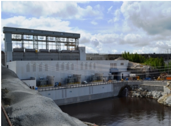
Photo 17 – View of the commissioned station now in service
