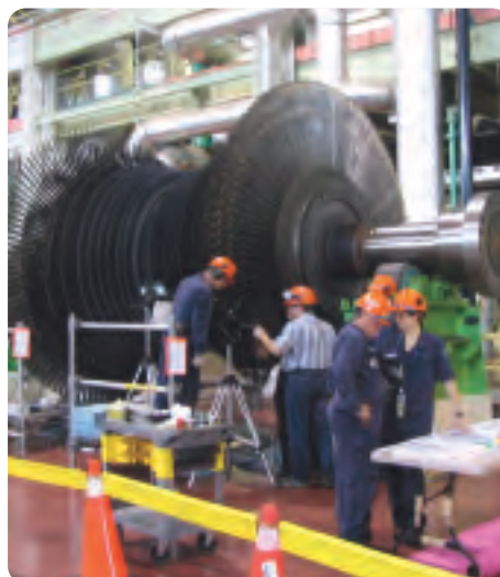
During the Pickering B Unit 7 outage, advanced ultrasonic technology was used to evaluate the condition of components of low pressure turbines.
