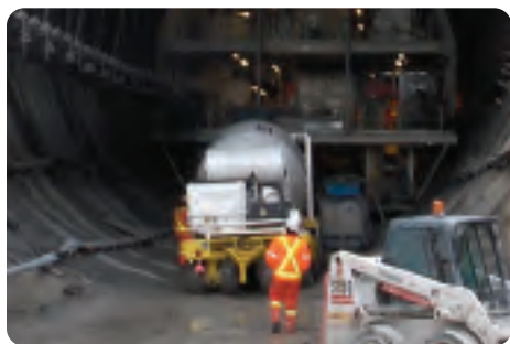
Big Becky, the world's largest hard rock tunnel boring machine, disappears from view as it proceeds to dig the Niagara Tunnel.
