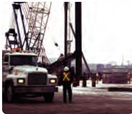
The Portlands Energy Centre will play a major role in supplying Toronto's energy needs.
