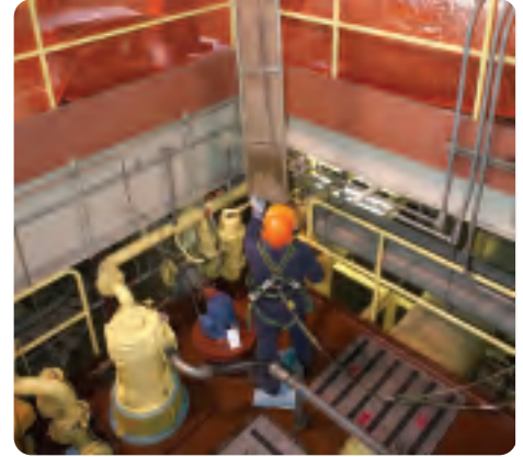
Pickering B employees performing outage work in 2006. OPG plans to make a recommendation on Pickering B's refurbishment to its Board early next year.
