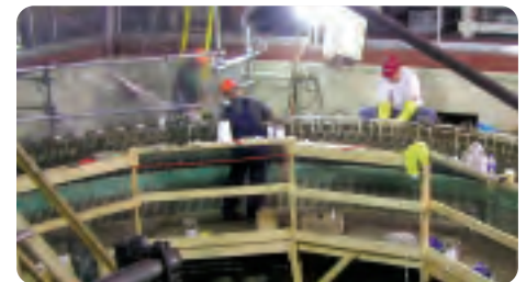
One of OPG Hydro's largest asset improvement projects, the Caribou Falls rehabilitation project involved staff from across OPG's Northwest Plant Group. OPG's hydroelectric assets have provided Ontario with clean, renewable electricity for many decades. Enhancements like these will help ensure they continue to produce for many years more.
