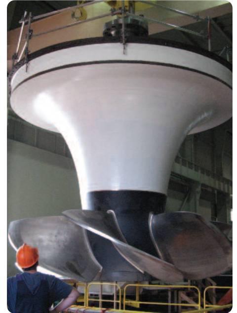
Equipment improvements like this runner replacement at OPG's Caribou Falls generating station helped add 12 MW to OPG's hydroelectric capacity in 2007.
