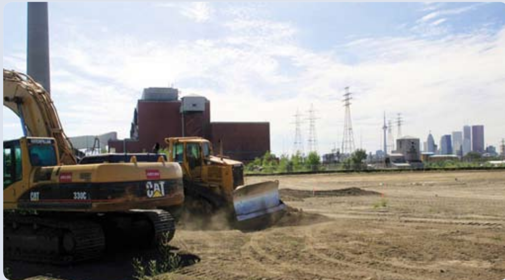
Site preparation for the Portlands Energy Centre, summer/fall 2006.
