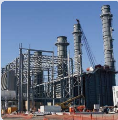
Structural steel on the main turbine building begins to take shape in the summer and fall of 2007.
