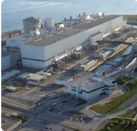
Darlington nuclear generating station in Clarington, Ontario
