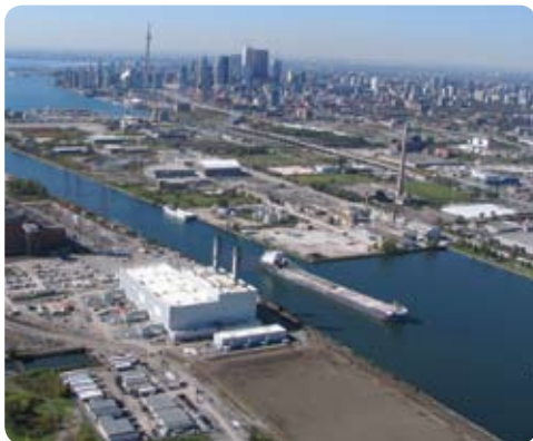
The Portlands Energy Centre helps serve Toronto's electricity needs.
