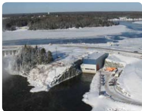
Lac Seul is OPG's newest hydro station, entering service in early 2009.
