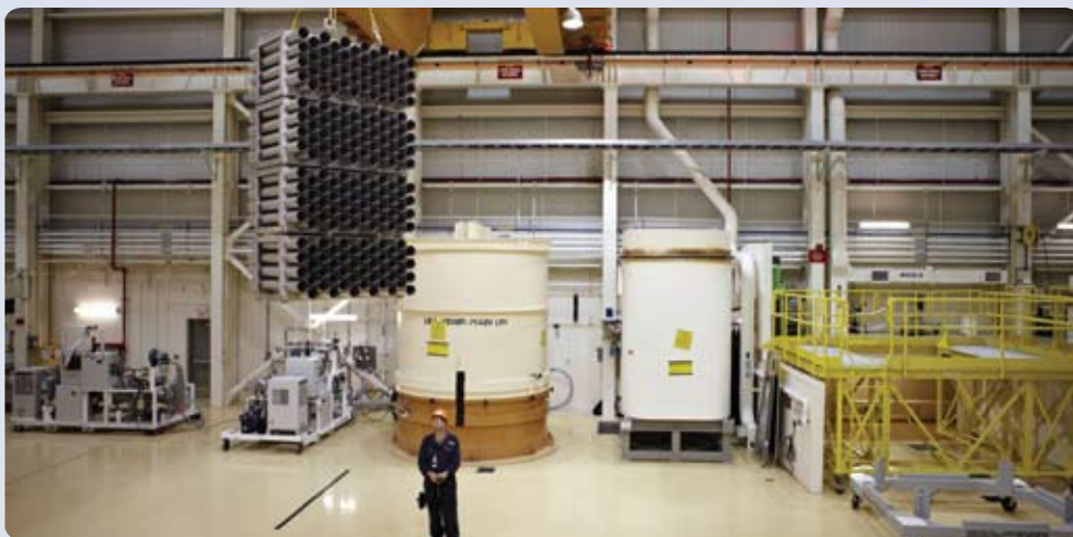
Darlington Nuclear Waste Management Facility
