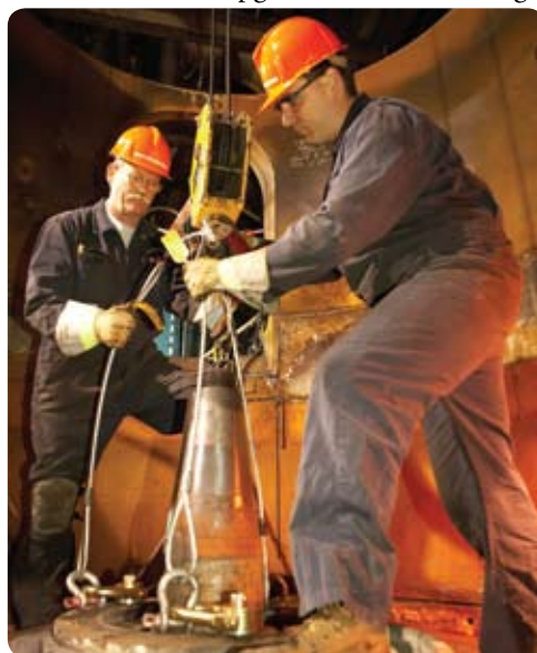
Lambton Unit 4 maintenance outage
