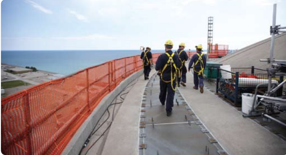
Outage staff on top of the Vacuum Building: To prepare for the outage, hoisting and rigging equipment were brought in, and a temporary elevator was erected to allow crews to access the roof.
