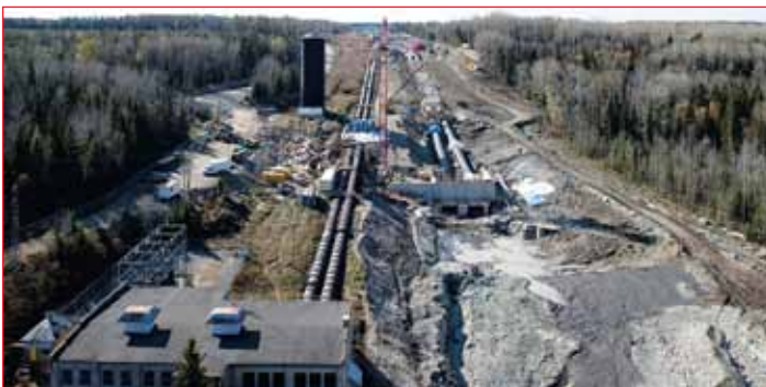
Construction of Wawaitin GS penstocks.
