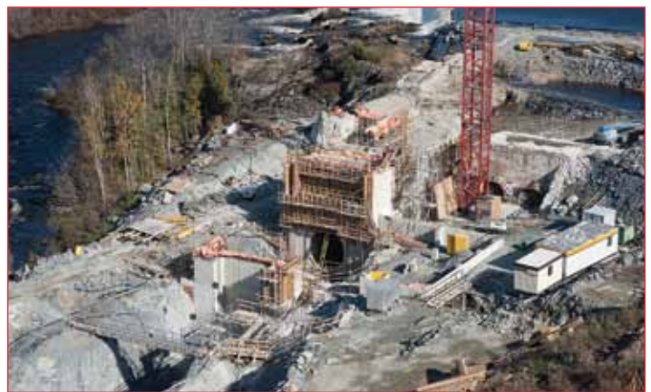
Construction of Sandy Falls intake structure, downstream.
