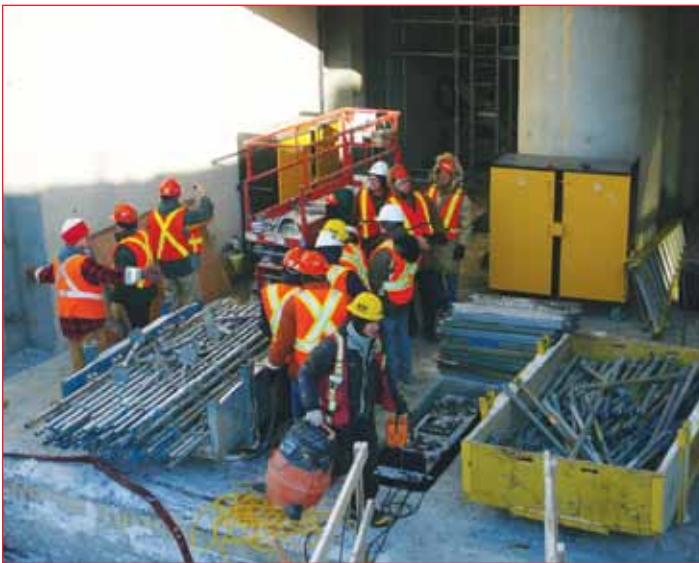
Construction workers at Wawaitin GS.
