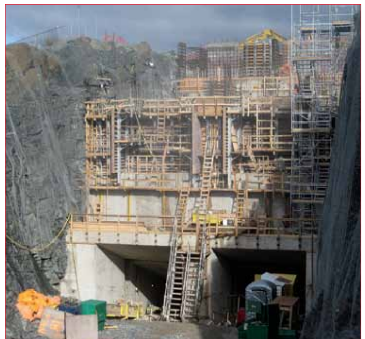
Close up of Hound Chute powerhouse under construction.
