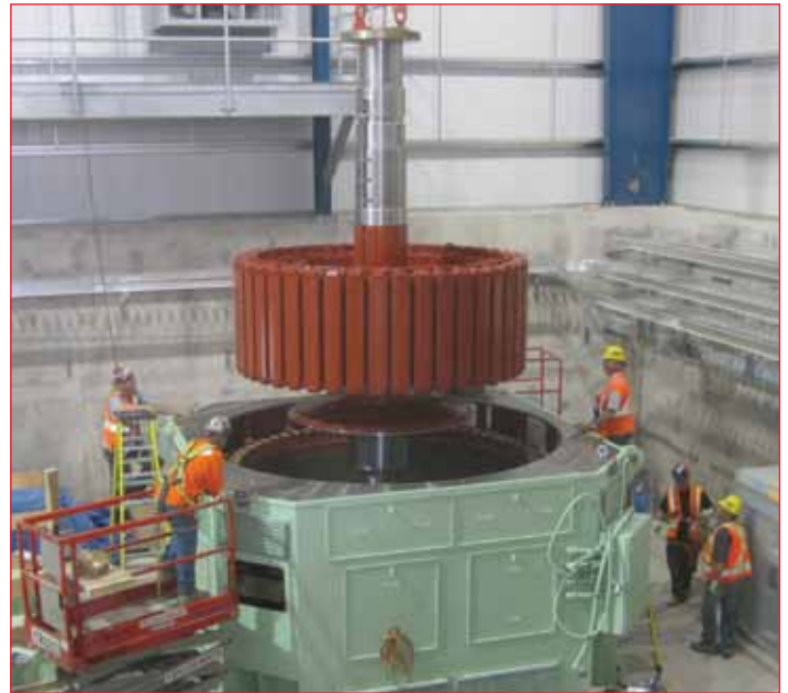
Lowering of rotor on Unit 2.
