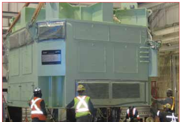
Installing new equipment at Sandy Falls.
