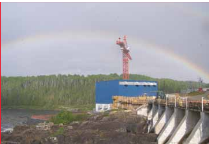
Lower Sturgeon GS powerhouse under construction.
