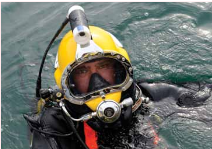
An OPG diver helps install OPG's protective fish net.
