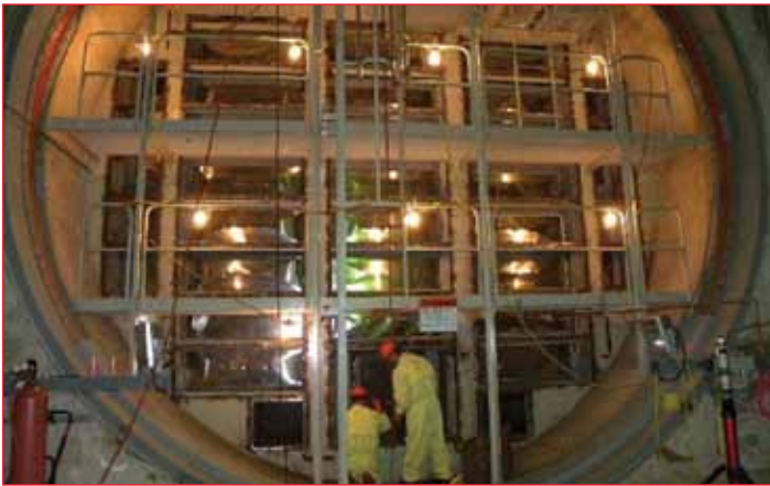
OPG staff work on the pressure relief duct bulkhead as part of the Safe Storage Project.
