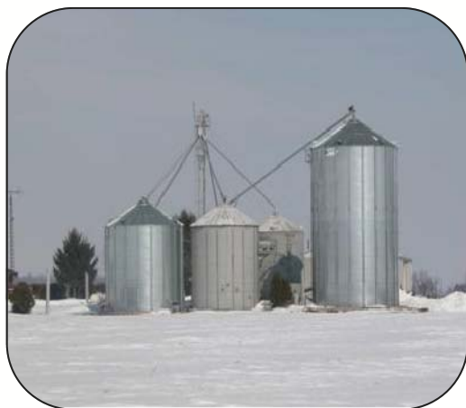
Figure 1. Successful grain storage requires routing inspection and aeration to avoid spoilage
