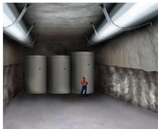
Intermediate level waste emplacement room
