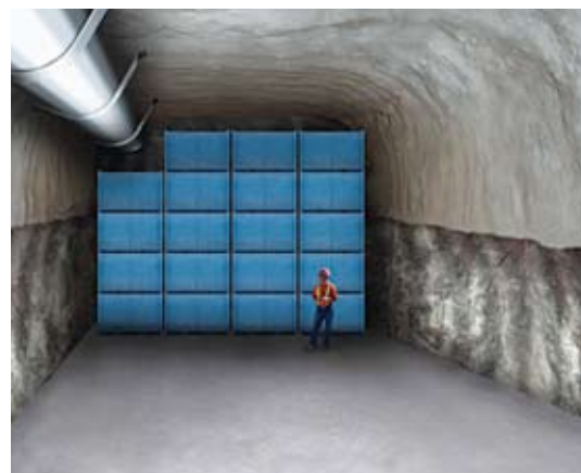
Low level waste emplacement room
