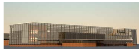
Queensway Carleton Hospital
