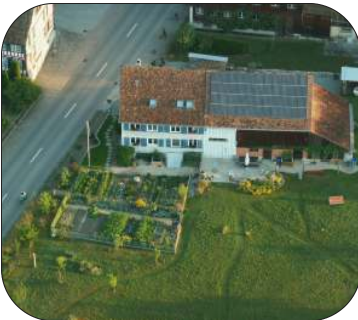
Figure 1. Solar photovoltaic installation on residence Hohentannen
