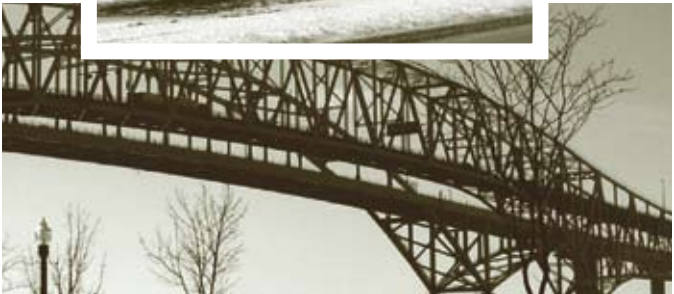
Bluewater Bridge, Sarnia ON
