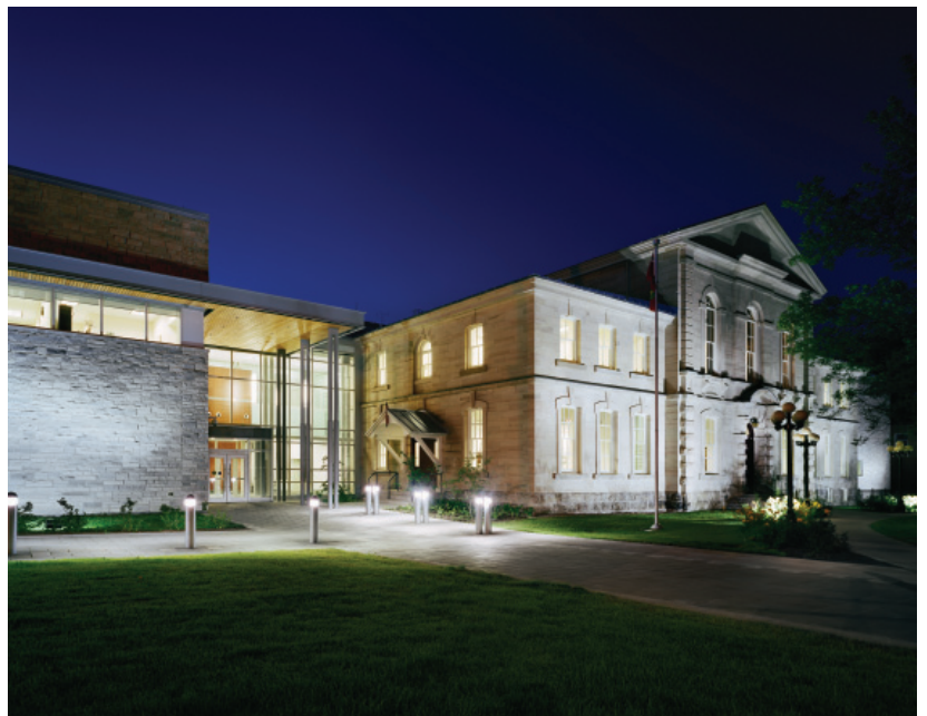
The New Renfrew County Courthouse
