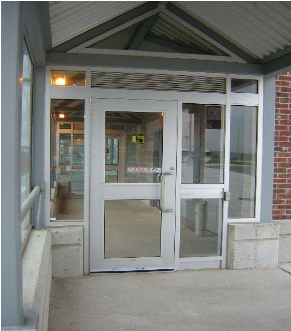
Example of a Wider Doorway
