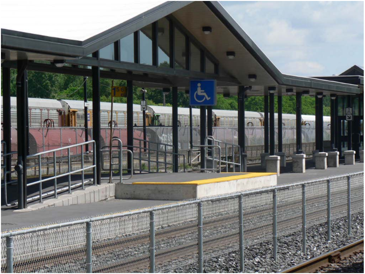
New Mini-Platform at Aldershot Station
