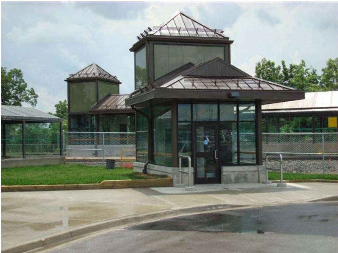
Tunnel Entrance Elevator at Erindale Station
