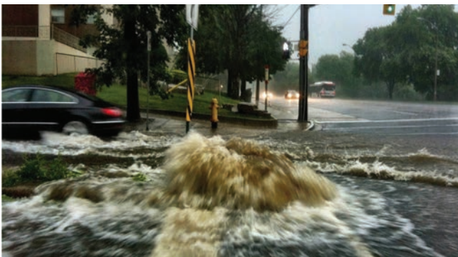
Flooding in the City of Toronto.
