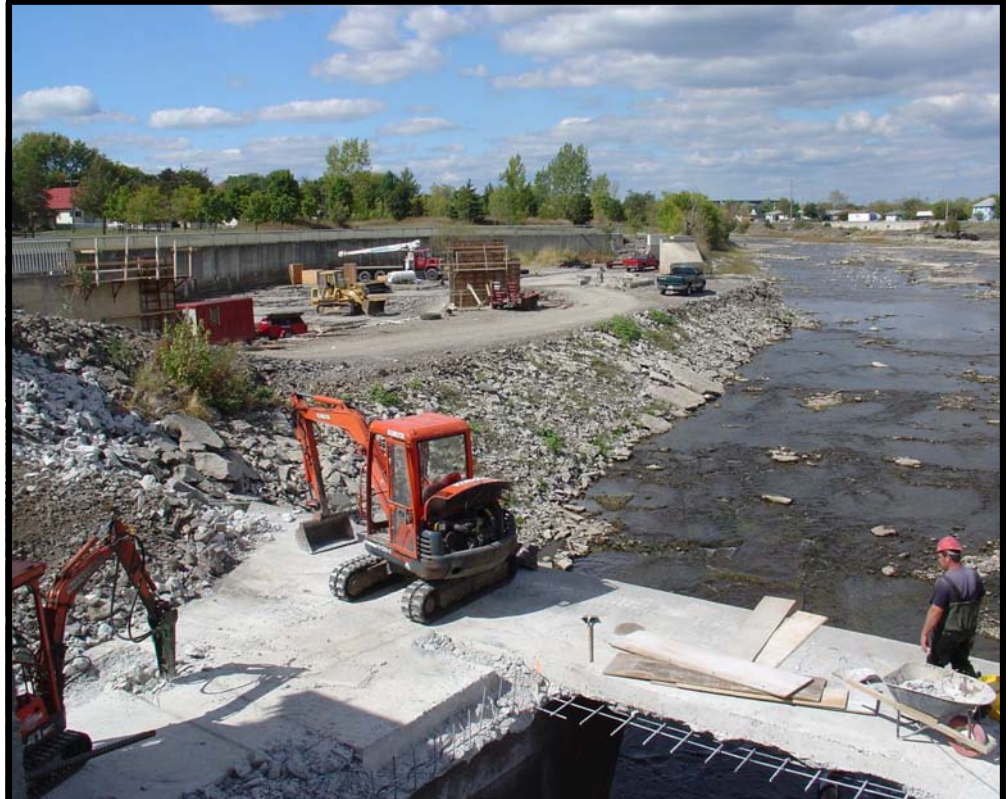
Construction on the Green Energy Project at the McLeod Dam in Belleville
