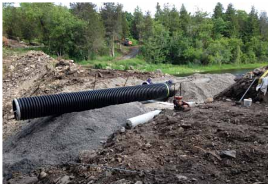
Harry Smith Dam during construction
