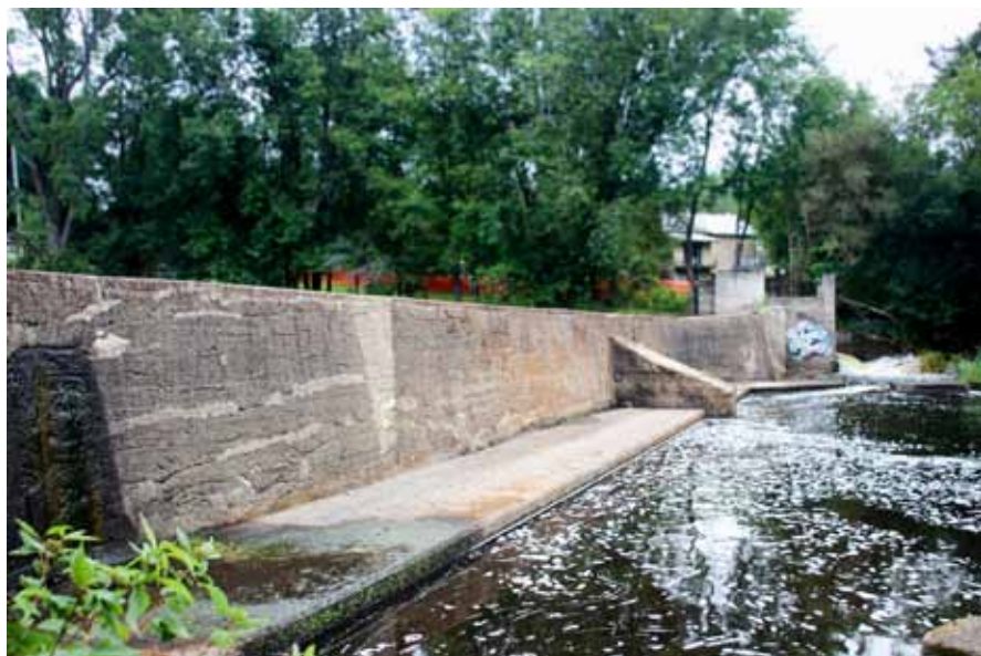
Colebrook Dam during construction
