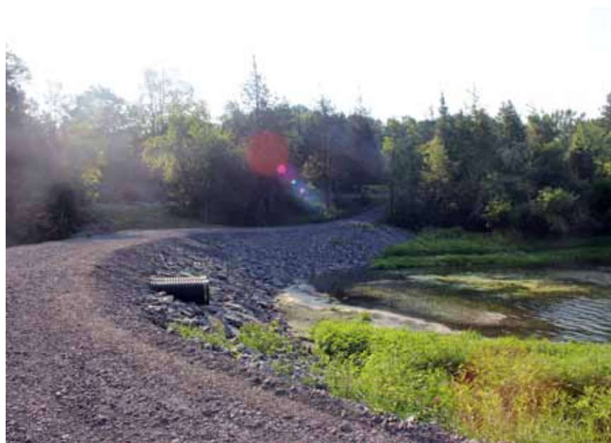
Completed work at Harry Smith Dam
