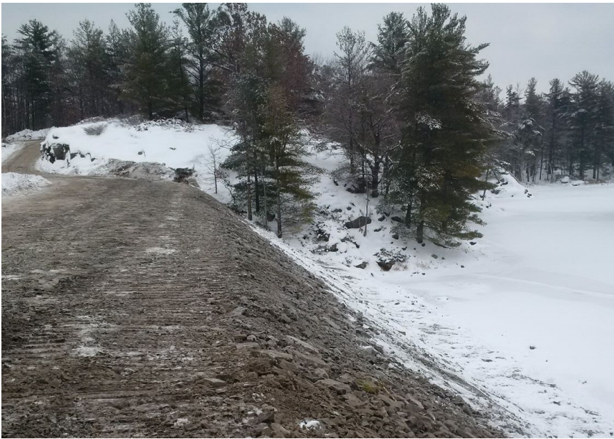
The dam at 3rd Depot Lake after phase 1 maintenance work was complete.
