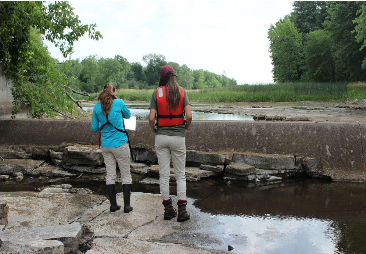
Water Resources Manager, Christine McClure (L), monitors the James Lazier Dam on the Salmon River during low water events in 2016.
