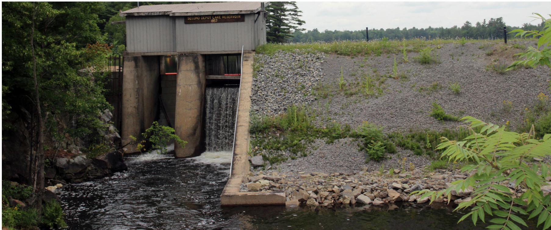
Dam at Second Depot Lake
