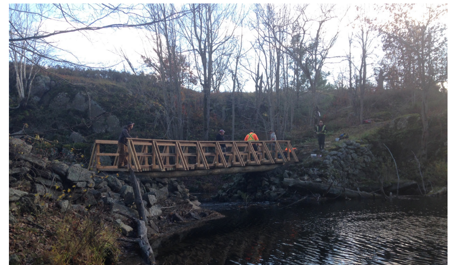
Workers replacing the bridge at Depot Lakes.
