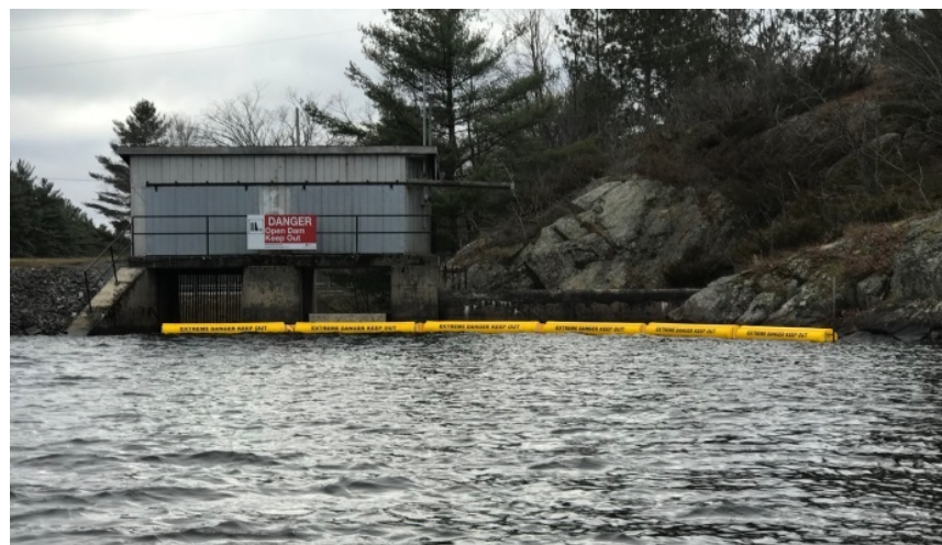
New booms at Second Depot Lake Dam
