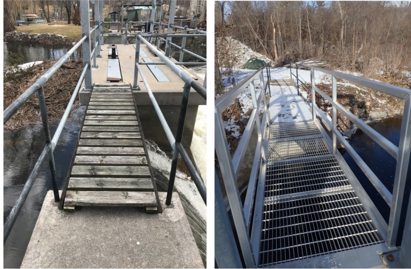
James Lazier Dam catwalk replacement
