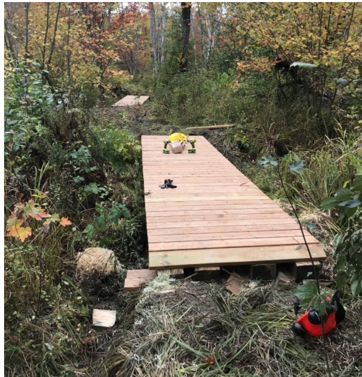
Newly constructed trail crossing at Lingham Lake Dam
