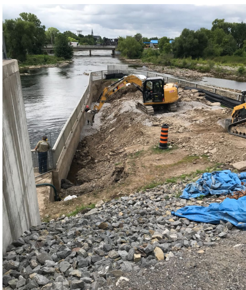
The beginning of placement of the pea stone and drainage tile. Picture taken looking downstream.
