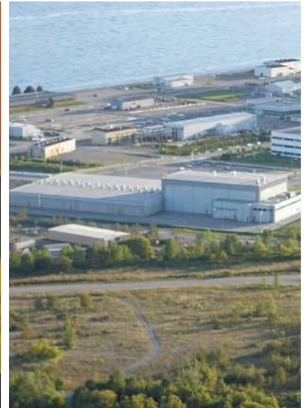
Darlington Used Fuel Facility
