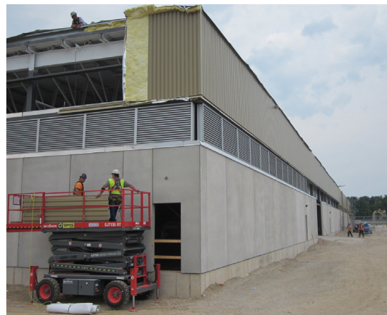
Construction of WWMF Storage Building
