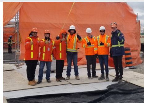
Pickering storage building foundation completed
