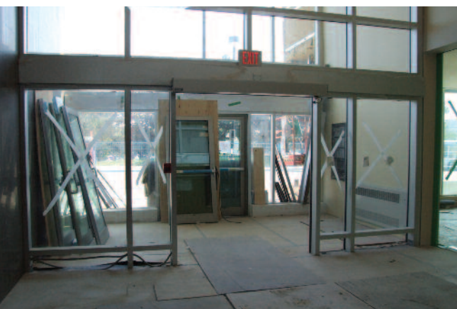
The entrance hall under construction.
