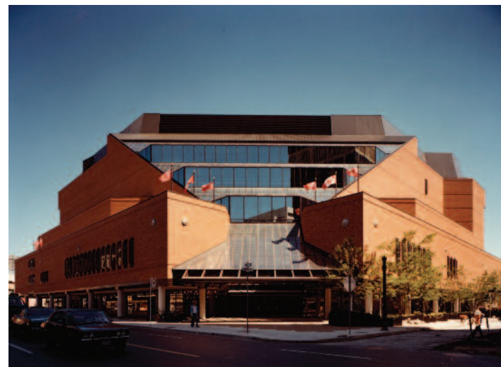
Metro Toronto Library - [Front entrance], 1973 Metro Toronto Reference Library by Moriyma and Teshima Architects and Planners / Archives of Ontario F 2187-1-20, 10040880 Photograph, colour.
