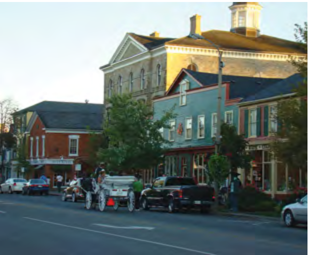
Niagara-on-the-Lake Heritage Conservation District
