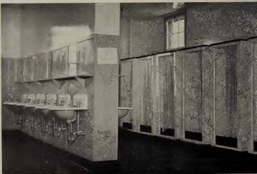
Showers and washroom, Rideau Industrial Farm
