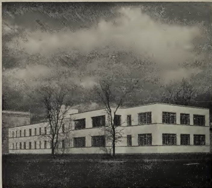
New Hospital Wing, Ontario Reformatory, Guelph.
