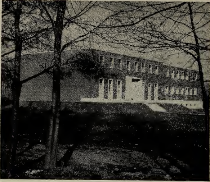
A new building—Hood House—opened during the year at the Ontario Training School for Girls, Galt.
