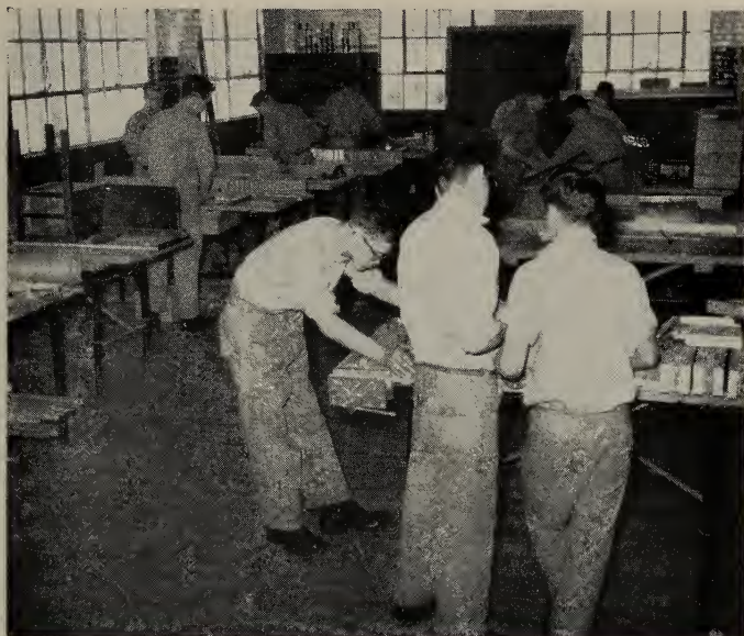
A section of the carpentry and woodworking shop at Bowmanville.
