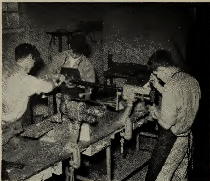
Vocational training is provided at the Guelph School— a section of the sheet metal shop.
