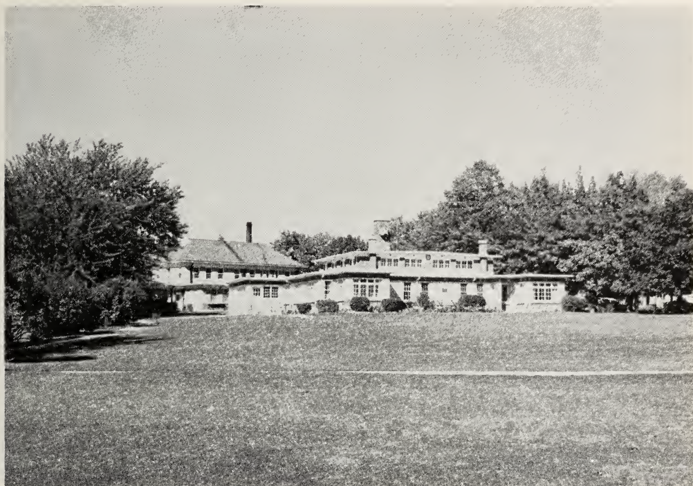
"Kiwaniis House" — Ontario Training School for Boys, Bowmanville.
