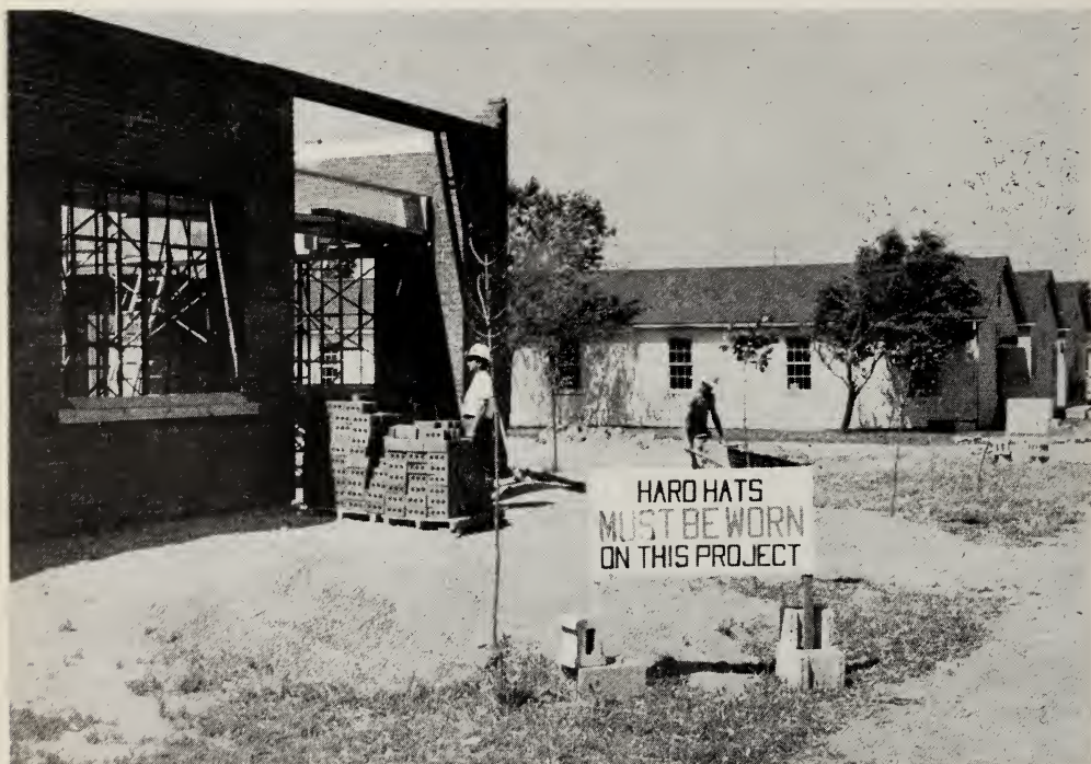
Auto-mechanics shop under construction, O.T.C. Brampton
