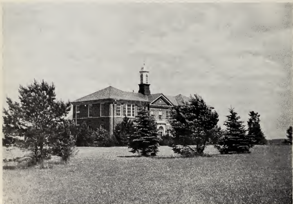
Administration and academic building, O.T.S. Galt.
