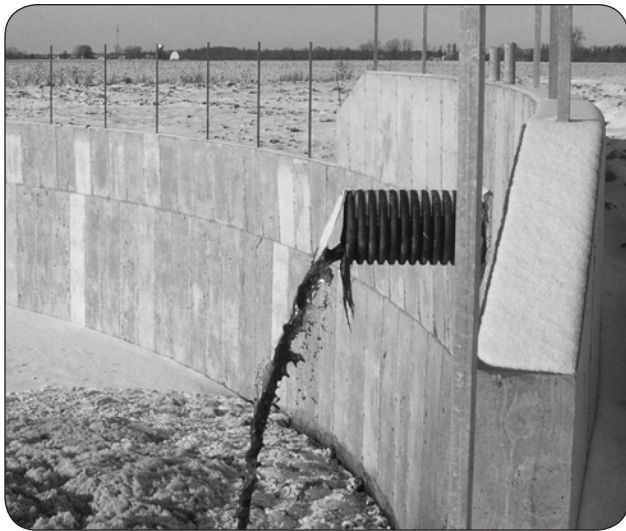
Figure 2. Gravity transfer system discharging over tank wall. Photo credit: Dietrich Engineering Limited
