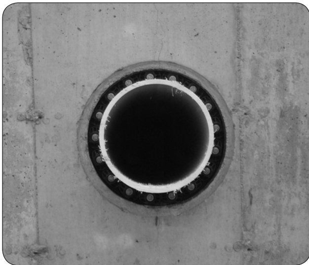
Figure 3. Modular seal through a concrete tank wall. Photo credit: Dietrich Engineering Limited
